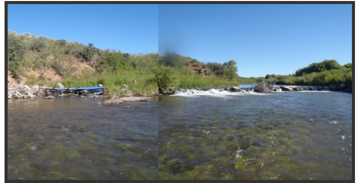
A diversion structure on the Smiths Fork River that is seasonally impassable by some species and sizes of fish
