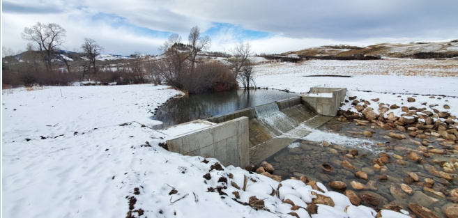
Figure 1. Fish barrier completed in 2019 on West Pass Creek to isolate Yellowstone Cutthroat Trout from other trout species.
