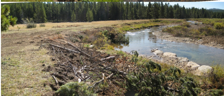
The active approach used at the Boy Scout site. The before (top left) shows eroding banks with a shallow stream depth. The after (bottom left) shows the use of woody debris, sod, and large boulders to stabilize the bank and deepen the river channel. At Dead Swede Campground (above), large boulders were placed to concentrate flow and stabilize stream banks.
