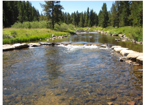
The active approach used at the Boy Scout site. The before (top left) shows eroding banks with a shallow stream depth. The after (bottom left) shows the use of woody debris, sod, and large boulders to stabilize the bank and deepen the river channel. At Dead Swede Campground (above), large boulders were placed to concentrate flow and stabilize stream banks.
