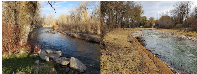
Figure 3. A recently installed beaver dam analog on Sourdough Creek west of Buffalo, WY.
