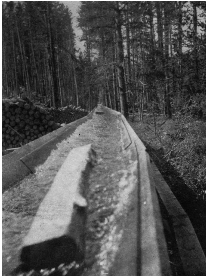
A tie flume used to transport rail ties from the Bighorns to Ranchester, WY.
