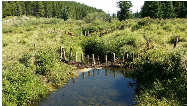
Figure 3. A recently installed beaver dam analog on Sourdough Creek west of Buffalo, WY.
