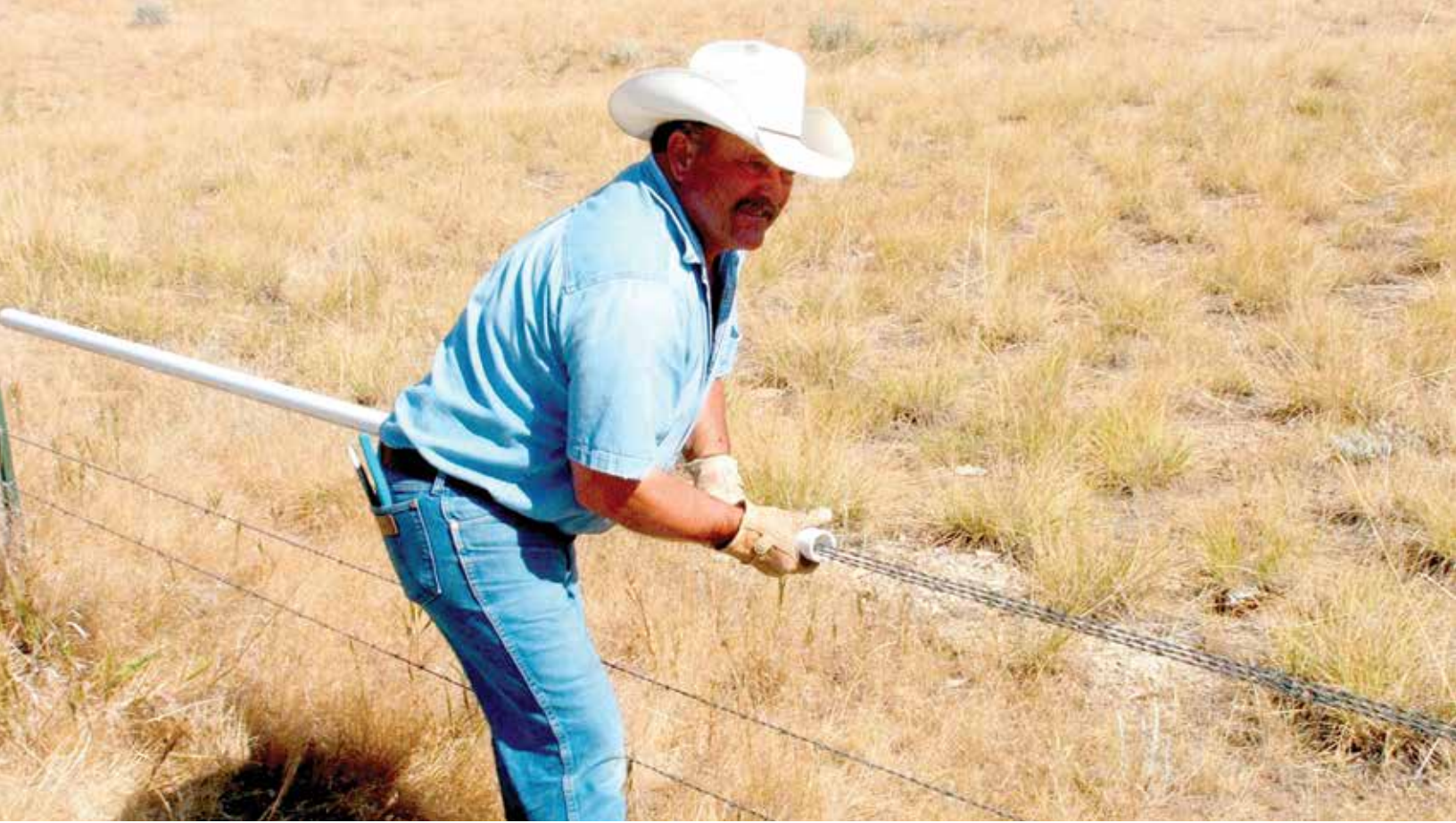
PVC pipe threaded over bunched fence wires and quick links to gather bottoms wires can create a durable big game passage, especially on road rights-of-way. Credit: Montana Fish, Wildlife and Parks.
