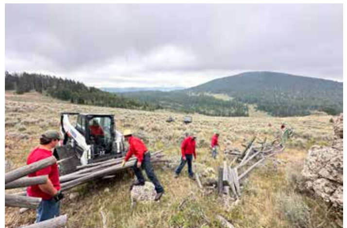
Cody Region Habitat & Access personnel removing buck and rail fence at Medicine Lodge WHMA.
