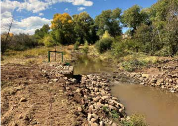
Natural channel design, fish friendly irrigation diversion at the Block diversion.
