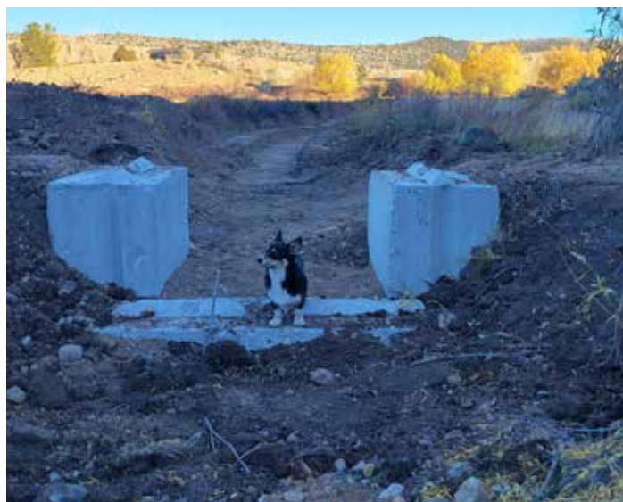
Check structure on the Whiskey Basin WHMA.
