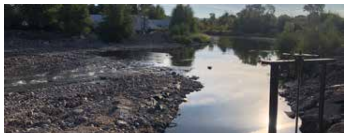
Sims Slough diversion after construction.
