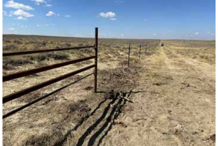
North Tipton Fence and crossing structure after removal of 23 miles of woven wire, and replacing with more wildlife friendly 4 wire barbed/barbless fencing.
