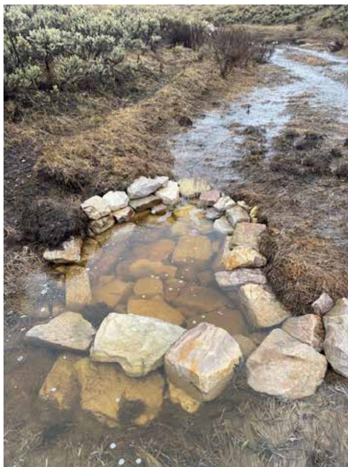
Zuni Bowl Constructed in Head-cut
