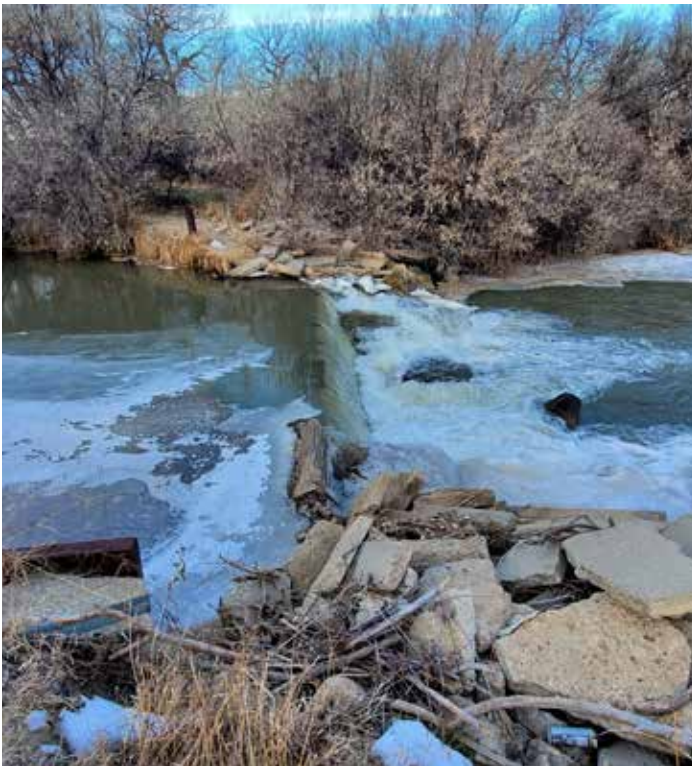
Modoc Diversion dam on the Middle Fork Powder River.
