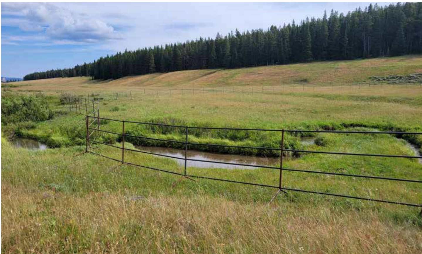
Steel Jack fence installed on upper Big Willow Creek.
