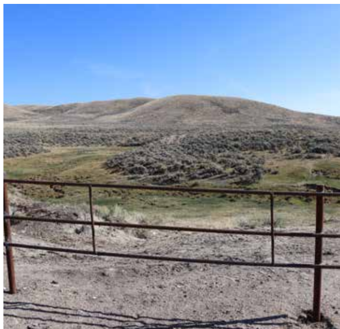
3-rail continuous panel pipe fencing protecting West Diamond Spring in the Diamond Springs Complex near Beaver Rim, north of Jeffrey City.
