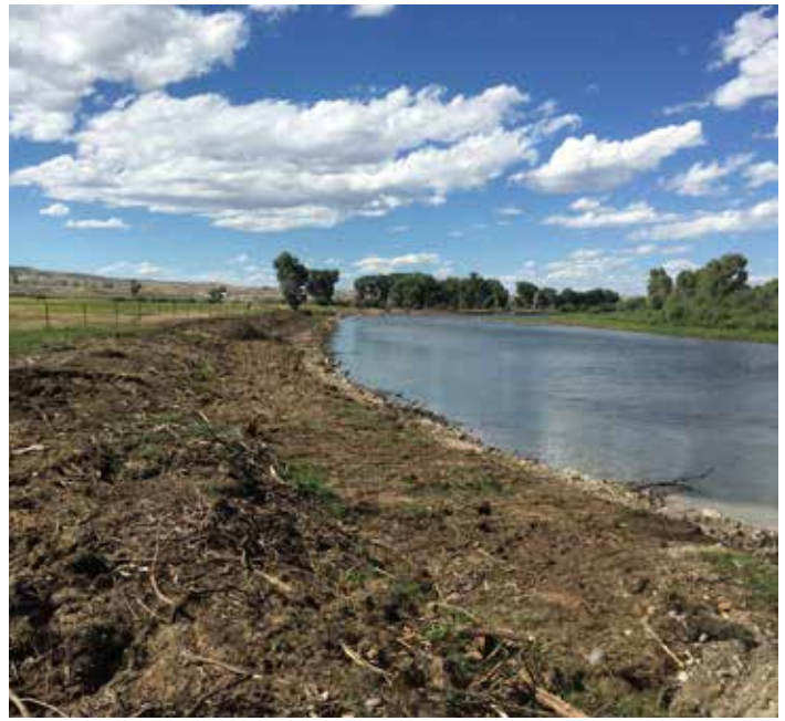
New Fork River bank stabilization.
