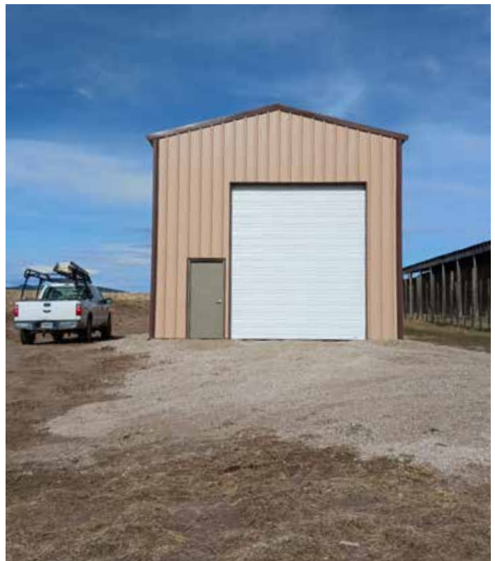
Insulated equipment storage -Black Butte Feedground.
