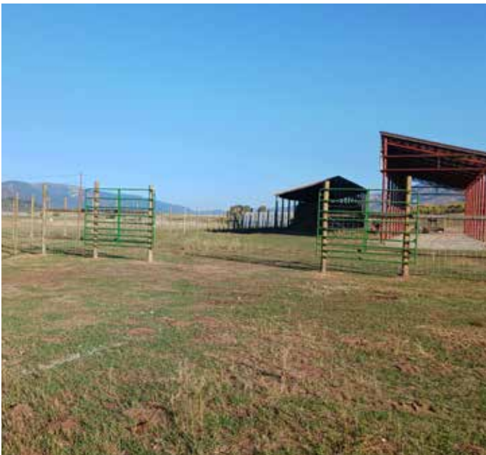
New 150' metal hayshed at the Alpine Feedground.
