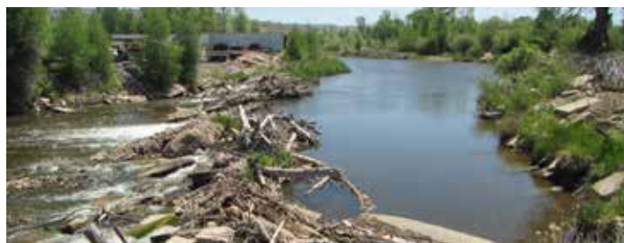
Sims Slough diversion before construction.
