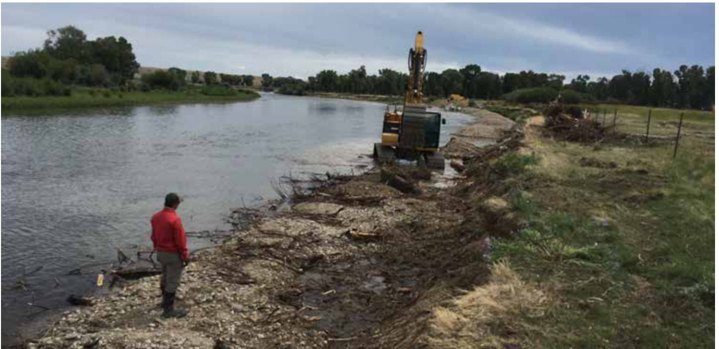
Construction of a bankfull bench at the New Fork River's Upper Olson work area.
