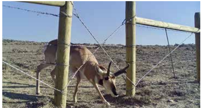
Buck pronghorn using newly installed X-gate crossing structure.
