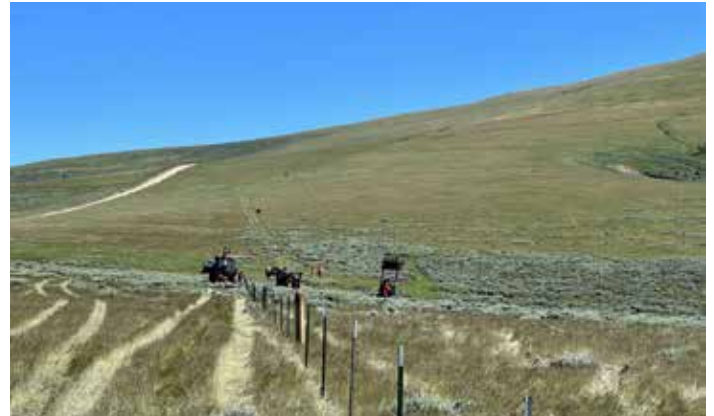
Parking and access development for the recently acquired Ellis WHMA.
