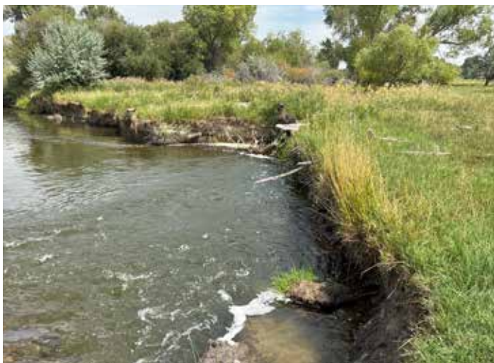
High water on eroding bank of Popo Agie River Country Garden state section.
