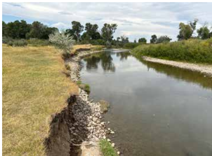
Bank erosion on the Popo Agie River Country Garden state section.
