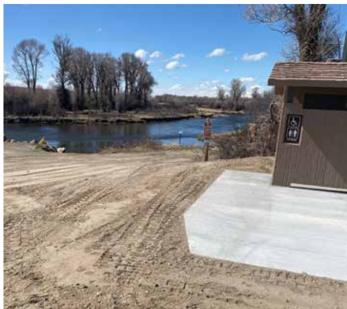
New comfort station and parking area New Fork Boulder Bridge.
