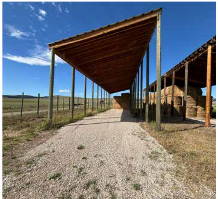
Road repairs and maintenance at the McNeel feedground 2024.
