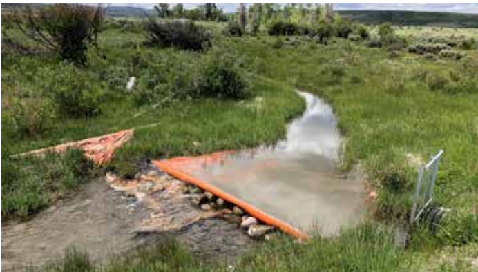
Diversion prior to construction.
