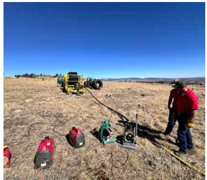
Poly pipe installation provides dispersed water options, Ed O. Taylor WHMA.
