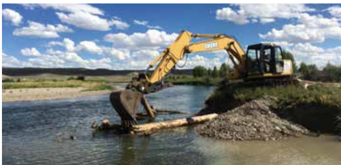
Construction of a woody jam on the Green River: Huston to Sommers Restoration.
