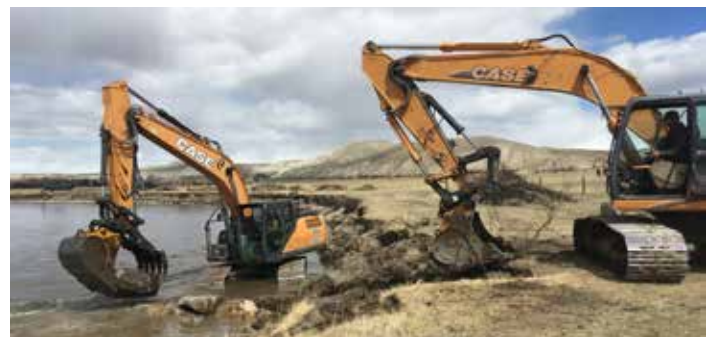
Construction of a woody jam on the Green River: Huston to Sommers Restoration.
