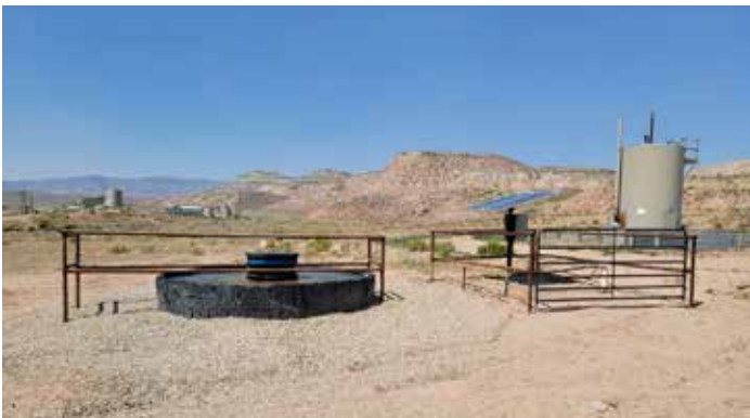
Chevron Well installation of a new solar array and tire tank.
