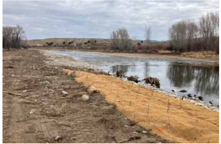
Bankfull bench constructed along the N. Platte River on the Kelley Place.
