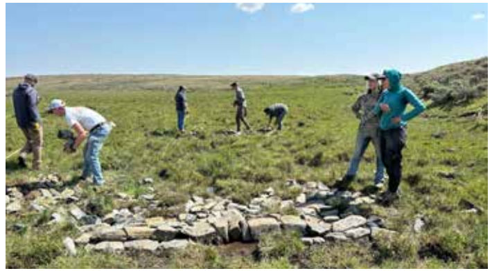
Installing a one rock dam Zeedyk structure on a Strawberry Creek tributary.
