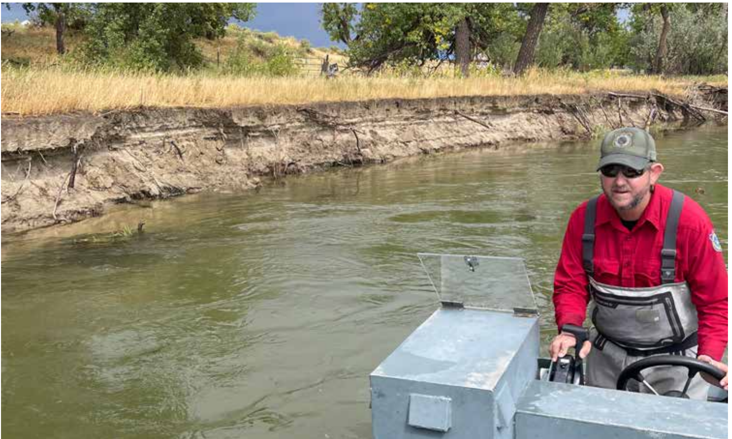
North Platte River North Platte Park eroding bank.
