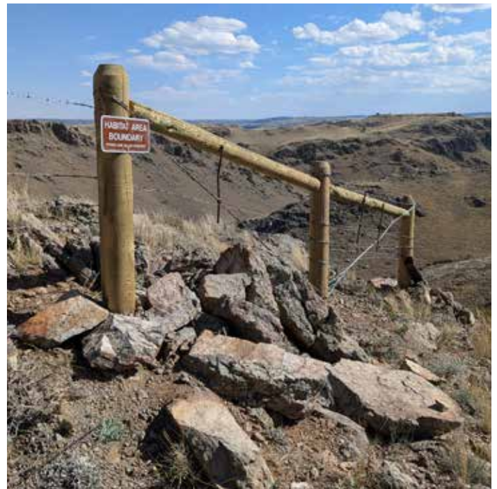
New wildlife friendly fence on Thorne Williams WHMA; Fellowship interns begin the process of removing overly tall woven fence and barbed wire in preparation for converting to four-strand.
