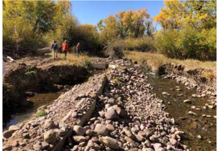
Block "Push-Up dam" irrigation diversion prior to construction.
