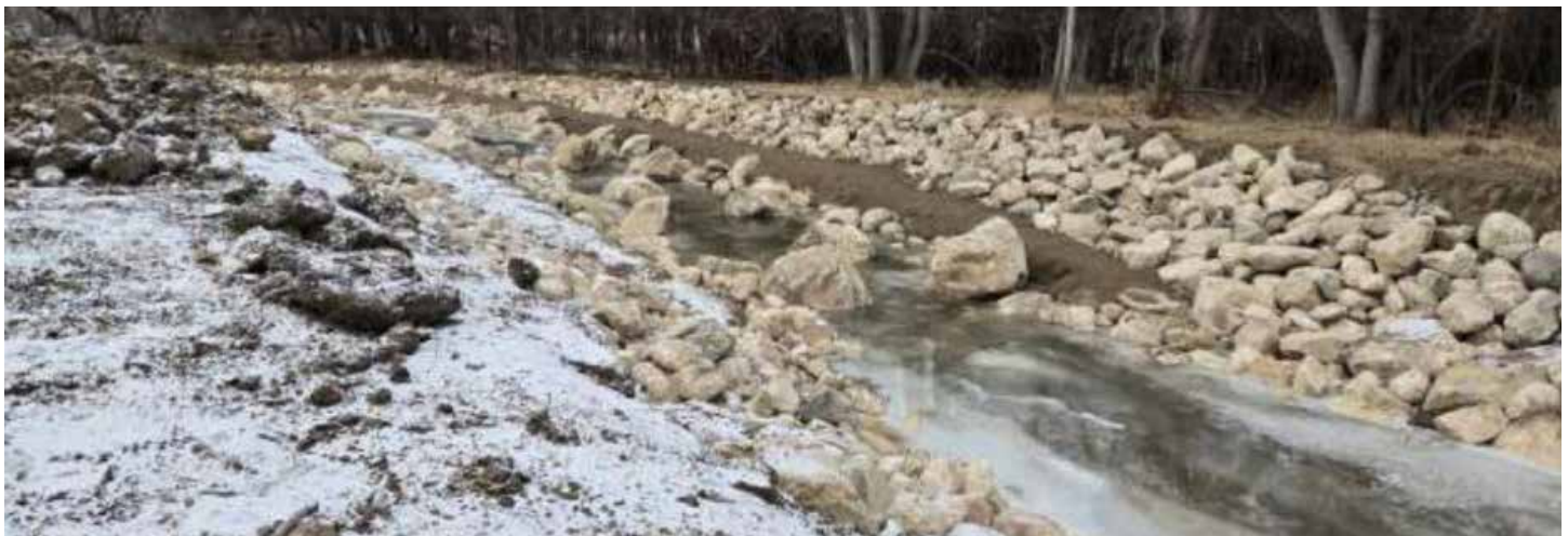
Fish passage ramp constructed downstream of the Downer Diversion on Soldier Creek (photo courtesy of the Sheridan County Conservation District).
