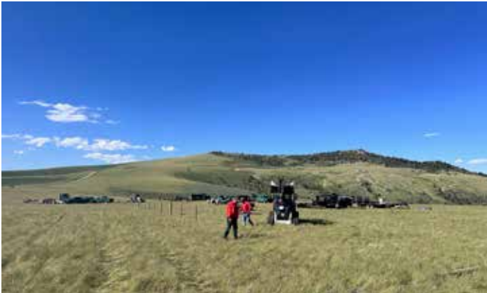
Parking and access development for the recently acquired Ellis WHMA.
