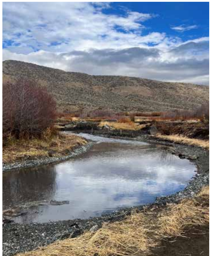
Completed bankfull bench and rock vanes to reduce erosion to the stream banks.
