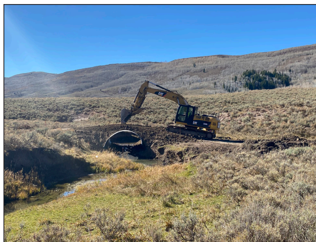
Figure 118. Bottomless arch installation.
