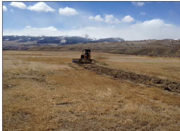
Figure 72. Clearing irrigation ditch on Bain Meadow.
