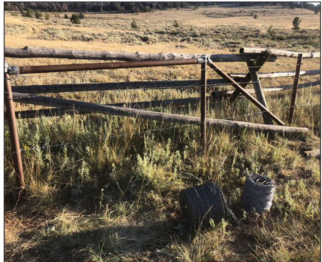
Figure 144. New fence construction on Ed O. Taylor WHMA.
