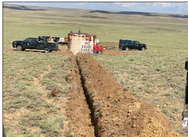
Figure 84. Installation of storage water tank.
