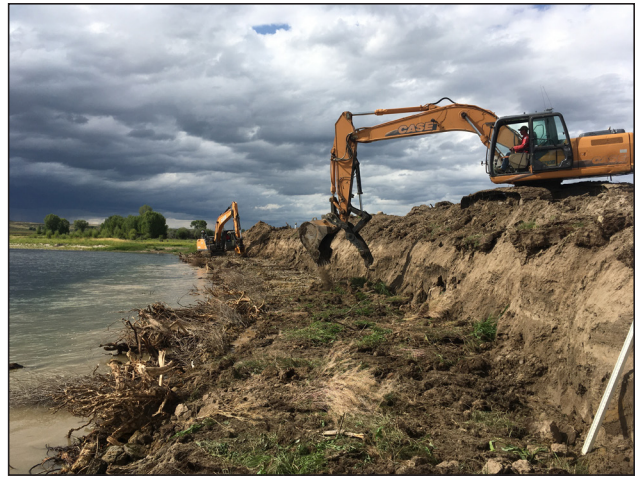
Figure 121. Bankfull bench construction on the Green River.
