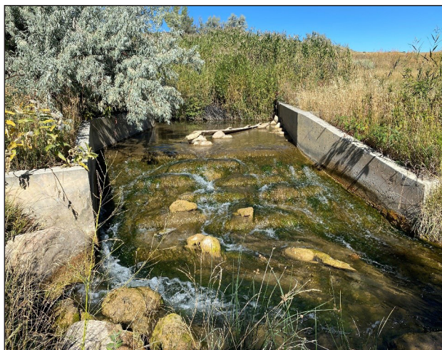
Figure 21. Paint Creek Falls diversion on Paint Creek.
