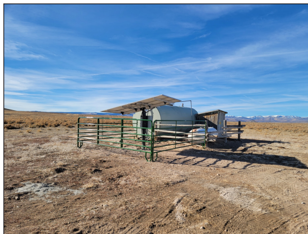
Figure 126. Installation of a solar array to power wells.
