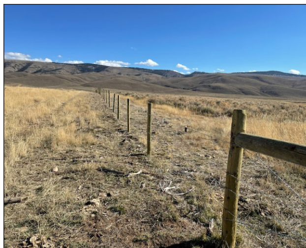
Figure 30. 4-wire wildlife friendly fence replaces netwire along mule deer migration path near Cokeville.
