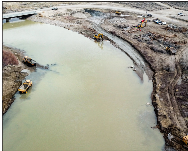
Figure 32. Green River urban restoration with crews installing live stakes.
