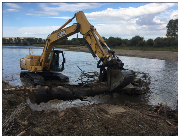
Figure 124. Rootwad installed at the Johnson Pasture.
