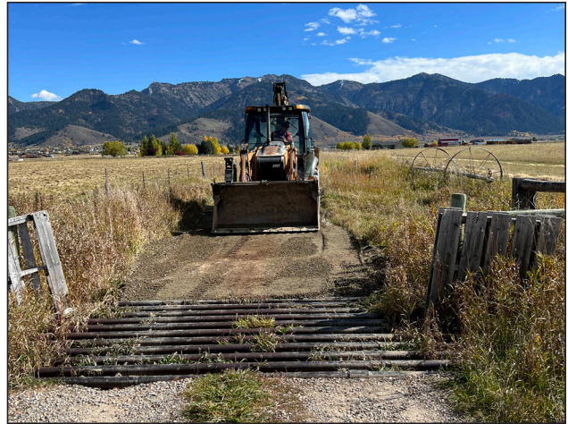
Figure 52. Road maintenance on Salt River PAAs.
