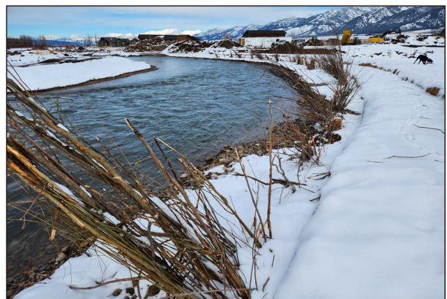
Figure 57. Recently installed toe wood, willow transplants and soil lifts.
