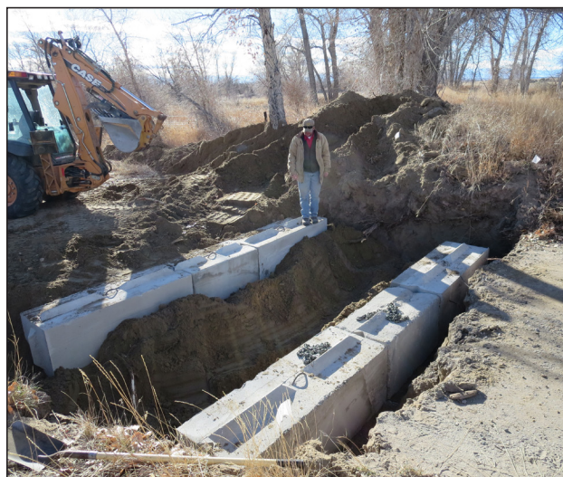
Figure 15. Installation of cattle guard base.
