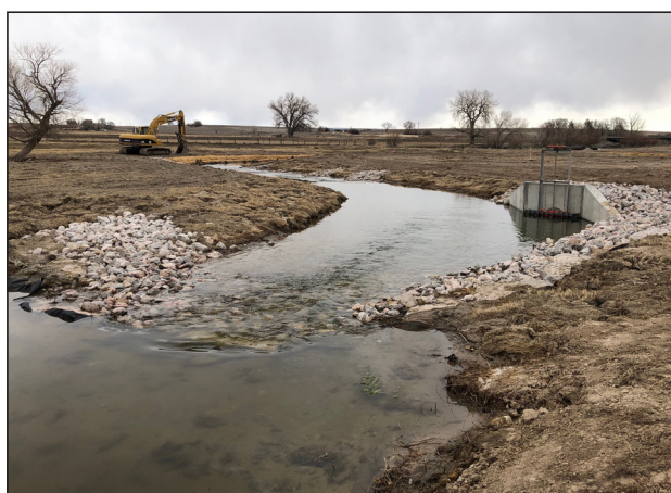
Figure 91. New Lawrence Ditch headgate on Horse Creek.
