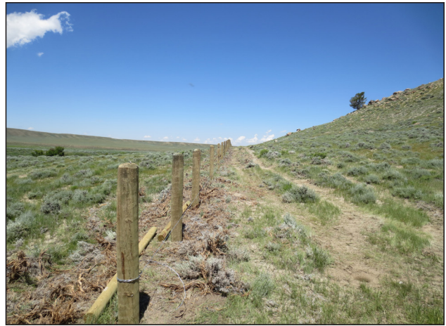
Figure 83. Willow Creek Fence under construction.
