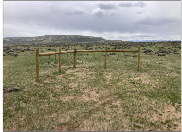
Figure 75. New corner brace on Spence and Moriarity WMA.
