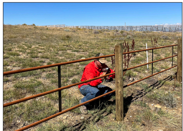
Figure 98. Wildlife friendly fence install.
