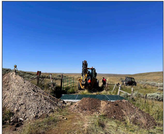
Figure 145. Cattleguard and gate installation on Ellis WHMA.
