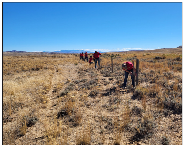
Figure 34. Converting highway ROW fence to wildlife friendly fence specifications.
