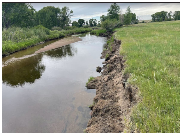
Figure 99. Typical eroding bank on the Laramie River.
