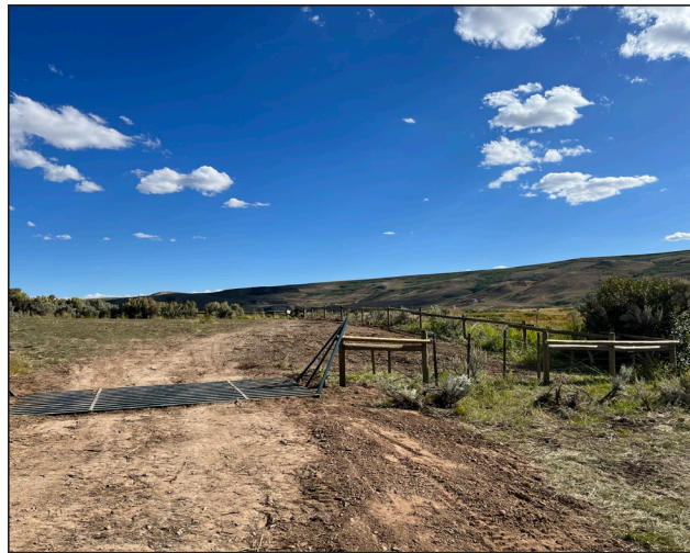
Figure 31. Hams Fork Bagley parking area fence conversion.
