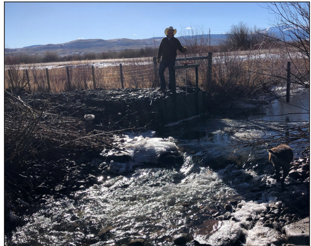
Figure 33. Natural channel design irrigation diversion on the Henry's Fork.
