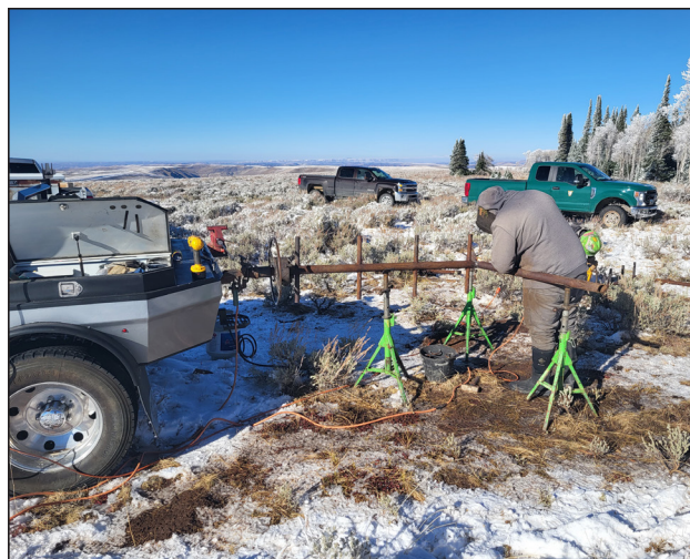
Figure 35. Repairing aspen enclosure fence on Little Mountain.
