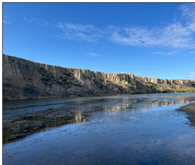
Figure 9. North Platte River Lusby eroding bank.
