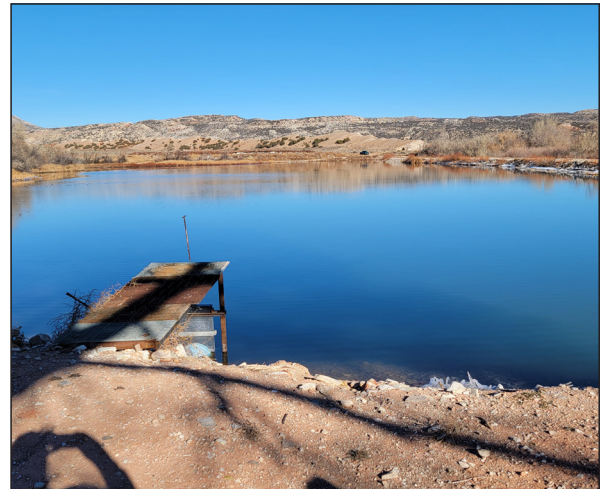
Figure 25. Tillett Springs rearing station post-completion.
