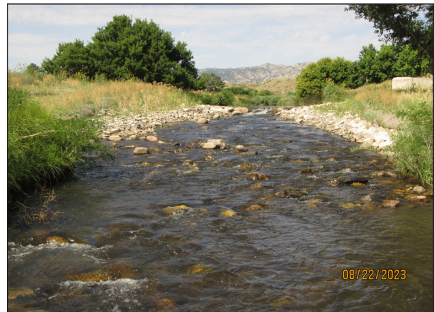
Figure 102. North Laramie River channel improved for fish passage.
