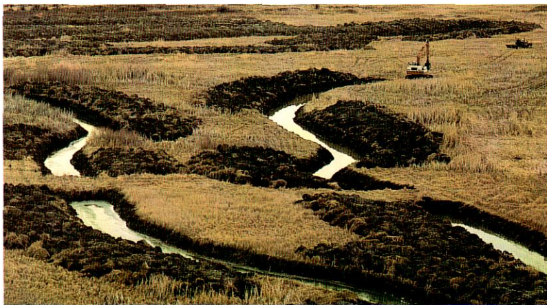
Where water tables are high, dredging or "level ditching" can produce wetlands with immediate benefits for water birds and many other wildlife species.
