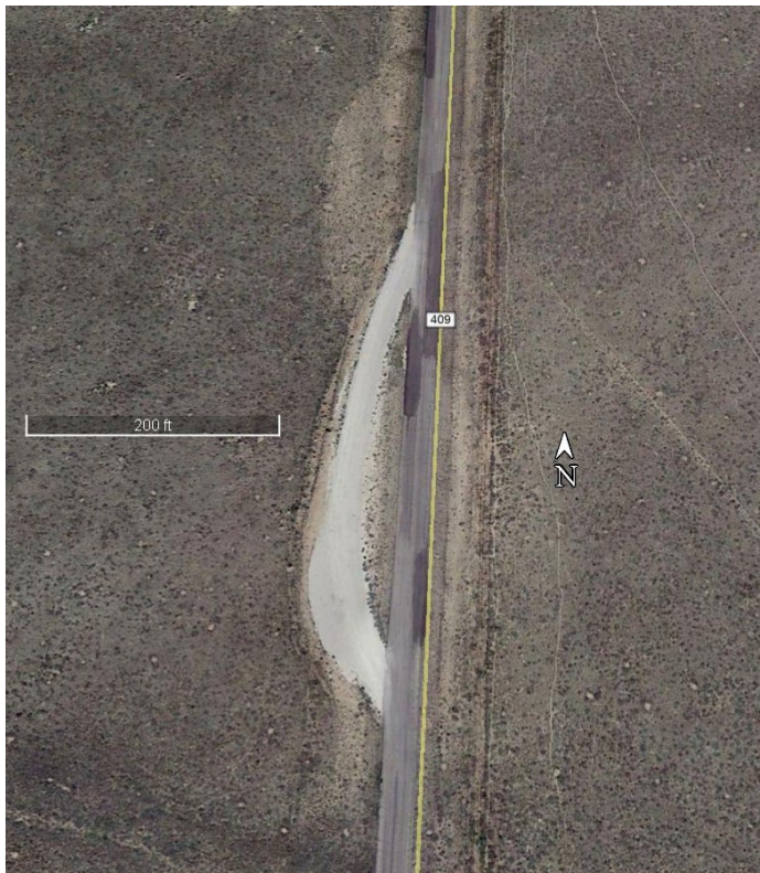
Figure 2. Aerial view of existing Pathfinder check station.
