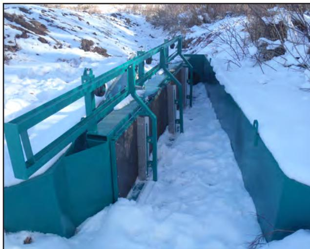
**Figure 4.** Vertical flat plate wiping screen that will prevent fish moving into the irrigation canal. The brushes move side to side wiping debris off the screen.
