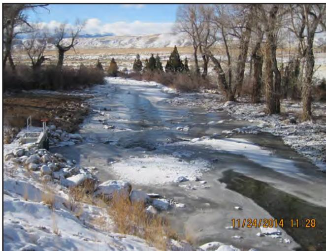
**Figure 3.** Bear Creek looking downstream with the head-gate on the left and four completed boulder cross-vanes in the channel below.
