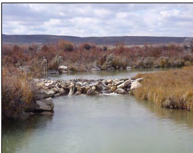
**Figure 5.** An instream diversion dam in the Cottonwood Creek drainage that is a fish passage barrier.
