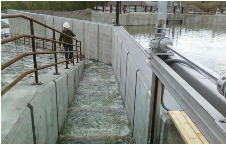
**Figure 5. The upper Sunshine Diversion fish ladder during post-construction testing in 2012.**
