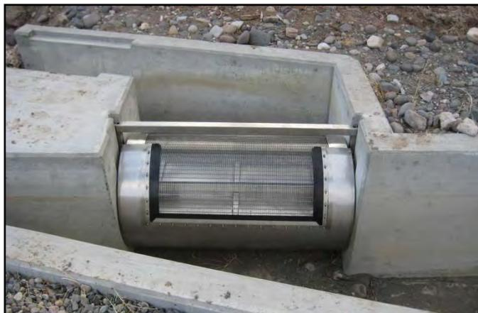
Figure 1. The Bear Creek fish screen was replaced with a larger screen of the same type when it was discovered that the ditch required more water than anticipated due to percolation and needed head to reach the end of the ditch.
