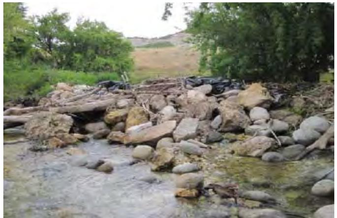
Figure 14. Irrigation diversion made of boulders, rock, and plastic. This fish barrier was removed and should be replaced with a more fish friendly structure in 2011.
