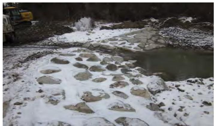
Figure 7. Post construction view of Bear Creek's downstream dam showing boulders with grout covered in snow, low flow channel in the middle, and the associated downstream pool. Stream flows are still diverted around the construction site in this photo.
