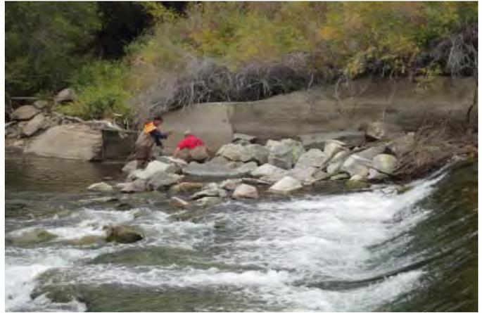
Figure 13. Fisheries biologist and consultant engineer evaluating the Encampment / Plate Valley Irrigation Diversion for potential installation of an upstream fish passage structure.
