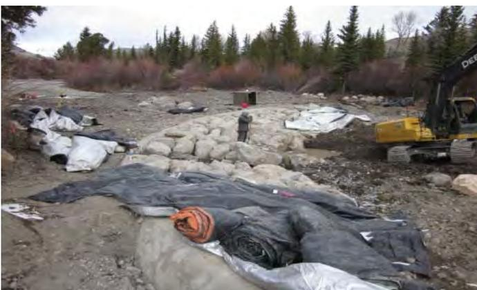
Figure 6. Bear Creek's upstream diversion dam under construction showing the low elevation concrete dam backed up by boulders which will be grouted into place and concrete blankets used to keep concrete warm while curing.
