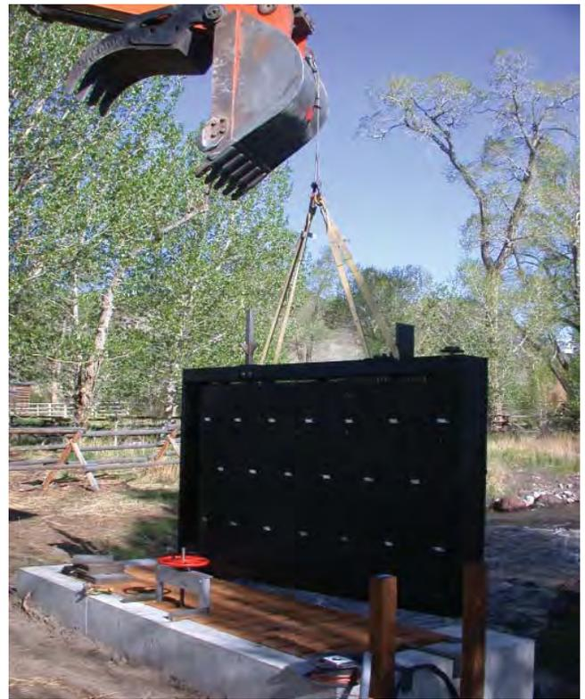
Figure 12. Reinstalling the traveling screen after modifications were complete.
