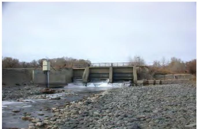
Figure 15. The Upper Sunshine Diversion Dam is tentatively scheduled for replacement in 2011. This structure is a barrier to upstream passage for Yellowstone cutthroat trout.
