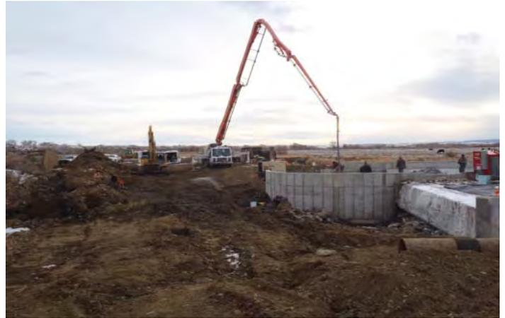
Figure 9. Concrete pump truck delivering concrete to the tall walls immediately below the box culvert and forming the curve that turns the fishway into the uplands, where it will curve in a horseshoe shape, gradually decreasing in elevation until returning to the creek.
