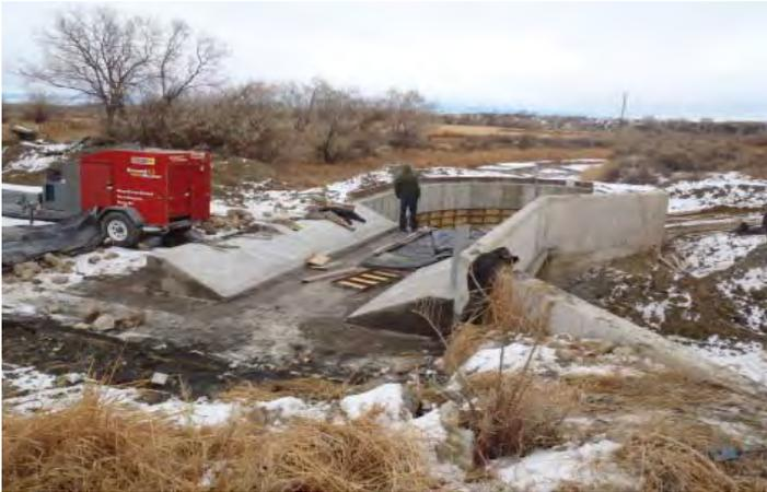
Figure 8. Upstream fishway walls formed at the right edge and on top of the concrete box culvert crossing Bitter Creek. The downstream curve will lead to the rest of the fishway when completed.
