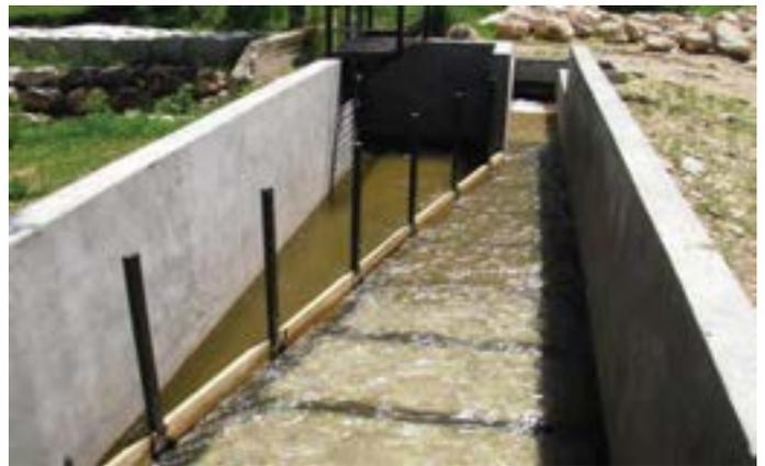
Figure 16. Screened fish from entering the diversion ditch via a flat bottom plate screen. The project reconnected 25.7-mile of the Tongue River downstream to the Interstate Diversion to 5.7-miles upstream to the York Diversion.
