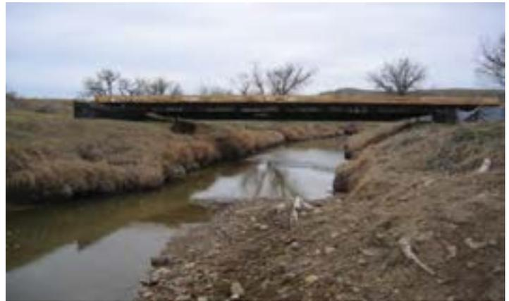
Figure 2. Crossing replaced with a full span bridge.
