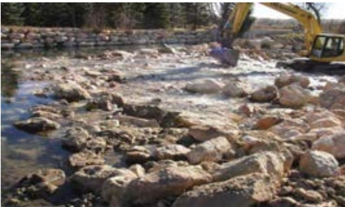
Figure 15. The Tongue River Diversion project provided fish passage over a roughened ramp.
