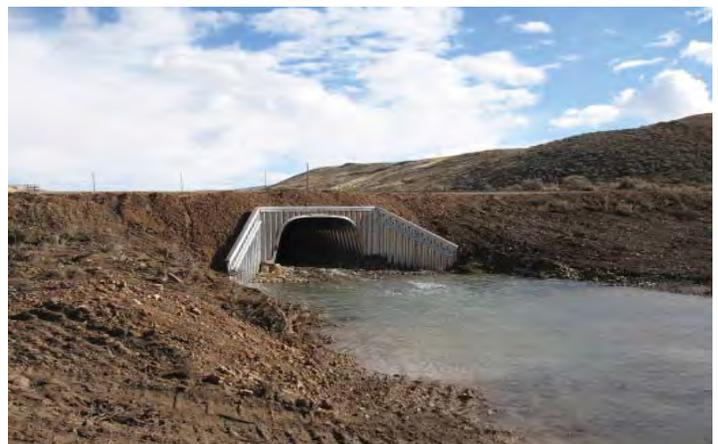
Figure 11. A bottomless arch-plate structure replaced the old culverts that were impeding fish movement on Twin Creek.
