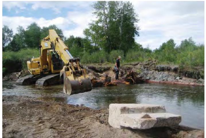
Figure 4. Vegetated riprap with rootwad spur habitat treatment along the Laramie River.
