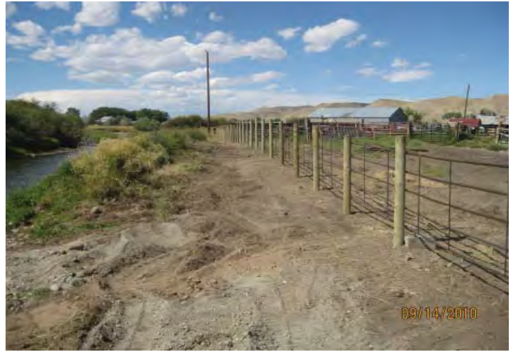
Figure 5. New fence along the corrals on the North Fork Popo Agie River eliminated a troublesome water gap.
