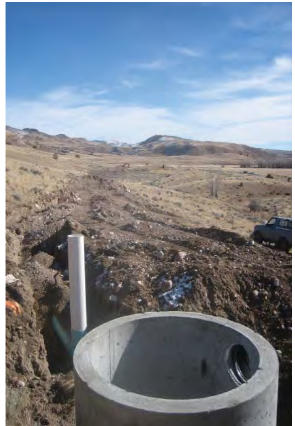
Figure 12. Pipeline and restoration on Dennison Meadows.
