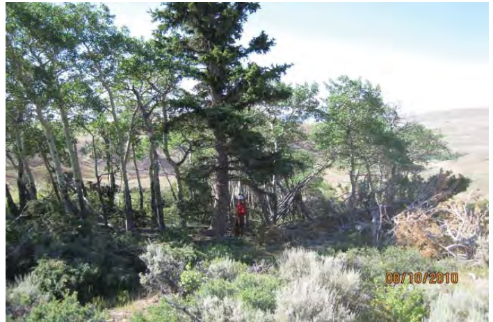
Figure 10. Crews removing conifers from aspen stands prior to fence construction.
