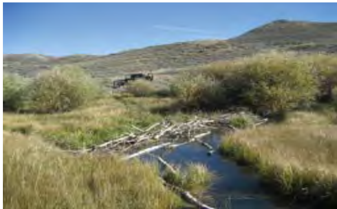
Figure 2. Supplemental aspen material placed for beaver to use in reinforcing and elevating the dam.
