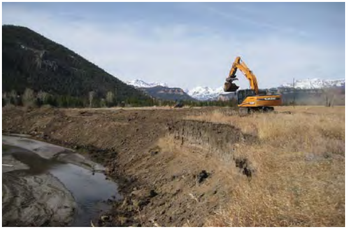
Figure 32. Stream bank stabilization at Sunlight Basin.
