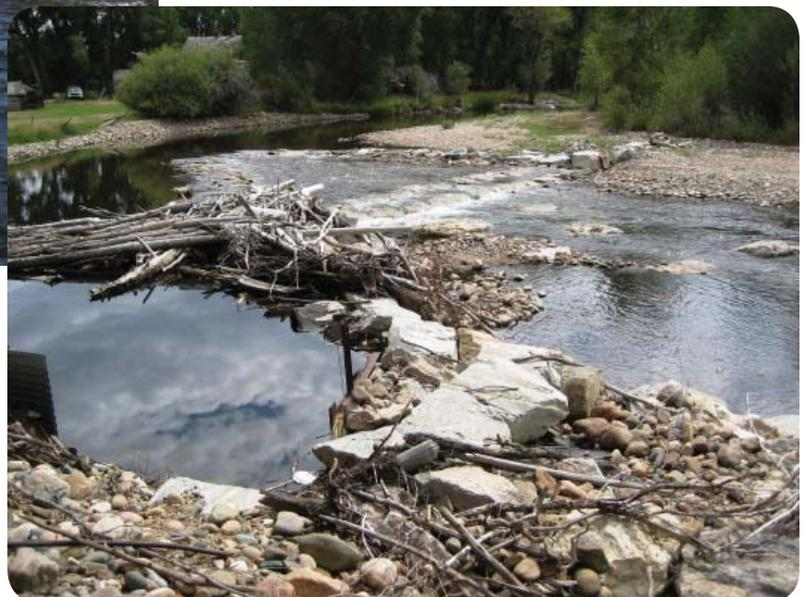
Figure 3. Cross-vane structure at an irrigation diversion at the upstream end of the Encampment River project area.
