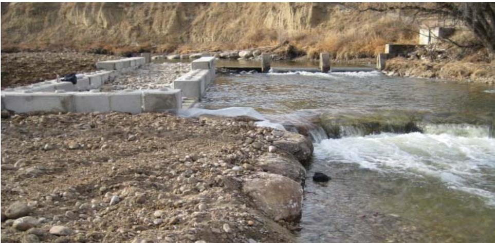
Figure 6. Rehabilitating the Big Bonanza Diversion on Clear Creek reconnected 16.4 miles of stream below the diversion to 3.1 miles of stream above the diversion. Work included vane structures and a rock ramp.
