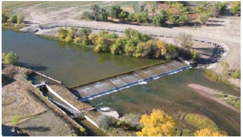
Figure 2. The T&Y Diversion bypass channel on the Tongue River south of Miles City, MT is the same design as proposed for the Tongue River and Clear Creek (MTFWP photo).
