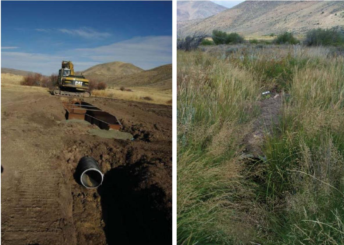
Figure 5a and Figure 5b. TU installed screen housings at 3 irrigation diversions on Rock Creek.
