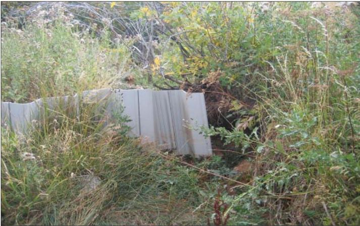
Figure 9. The riparian structure prior to repair looking upstream; the stream channel had washed out around the right edge.
