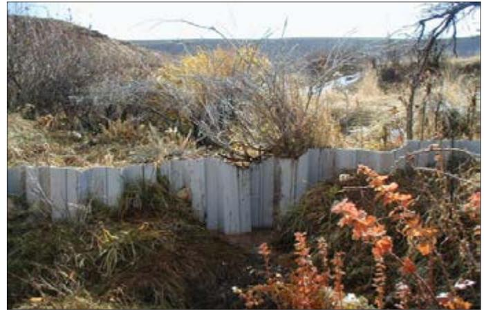
Figure 10. The structure after extending the sheet piling across the stream channel.
