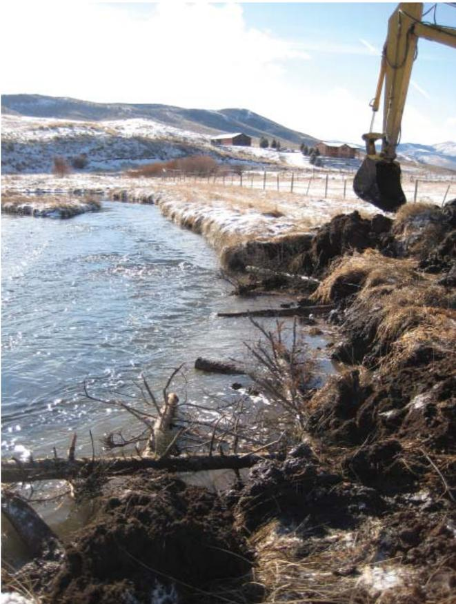
Figure 7. Placement of tree revetment structure on upper Crow Creek.
