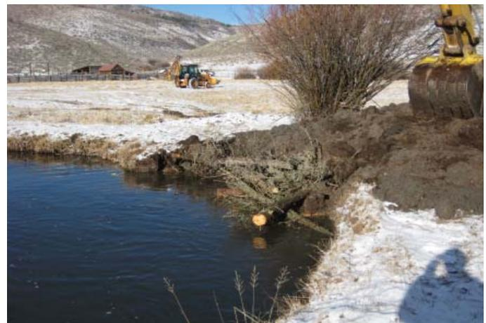
Figure 8. Tree revetment structure in a jackstraw formation.
