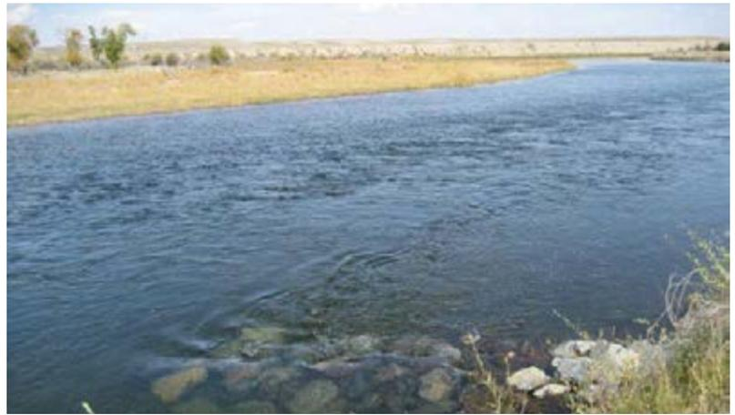
Figure 4. Completed rock barb jetty structure slowing river thalweg velocities, providing rock structure with niche habitat, and scouring attractive pool habitat for fish.
