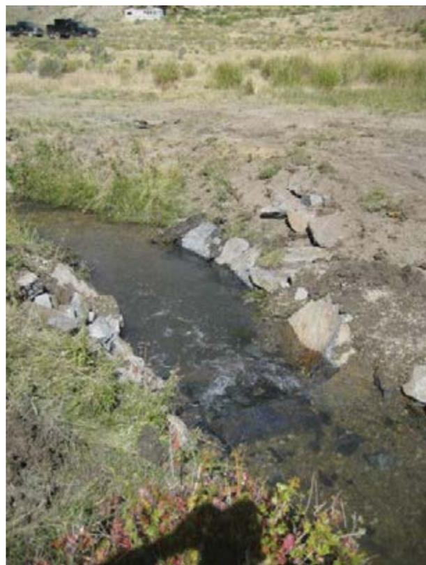
Figure 8. Completed rock weir structure in Currant Creek serving to control grade for restoring riparian meadow habitat and provide a pool for trout.
