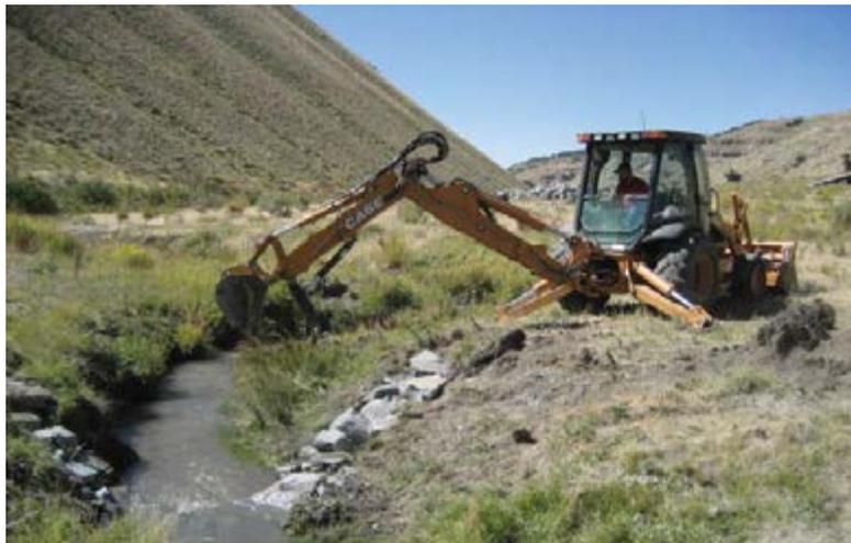
Figure 7. Statewide Habitat and Access Maintenance personnel constructing a rock weir gradient control structure in Currant Creek.
