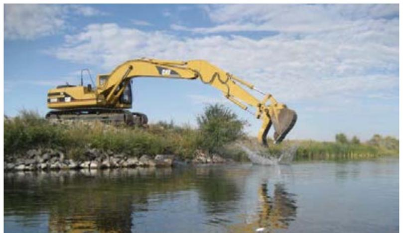
Figure 3. Seedskadee NWR personnel constructing a rock barb jetty structure in a reach of the lower Green River to improve fish habitat.
