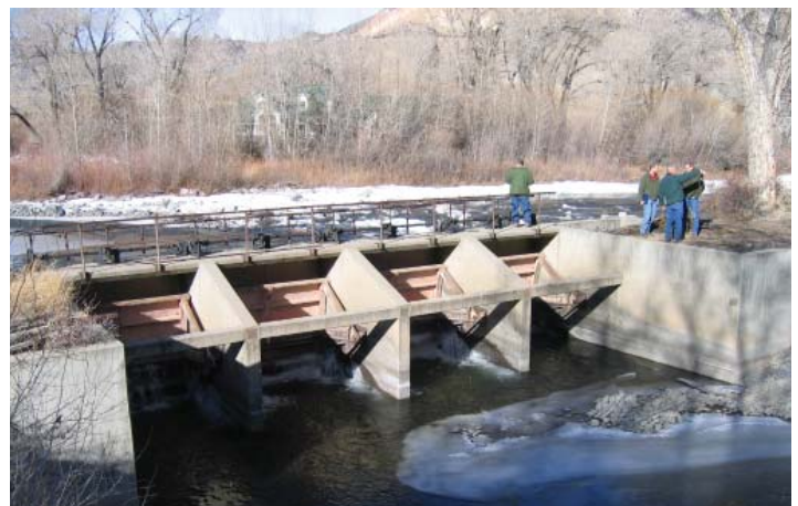
Figure 8. Cody Canal Irrigation Diversion on the South Fork Shoshone River near Cody.
