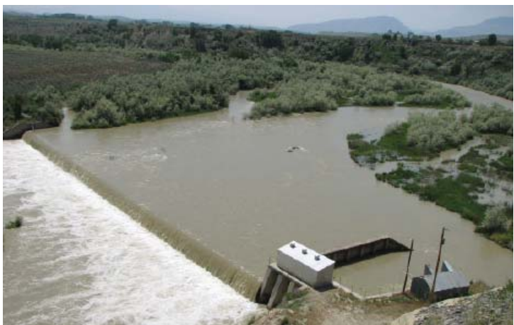
Figure 7. Corbett Dam on the Lower Shoshone River near Cody.
