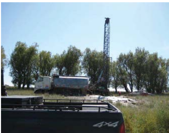
Figure 21. Wellnitz Ponds well drilling
