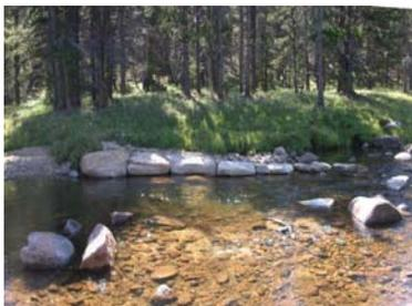
A bank stabilization structure preventing bank erosion while creating fish habitat.
