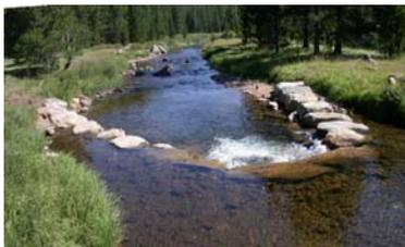
A "cross vane" structure concentrates the flow towards the middle of the channel which helps to alleviate bank erosion but also provides pool habitat for fish.
