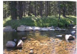
A bank stabilization structure is used to prevent bank erosion while also helping to create pool habitat.
