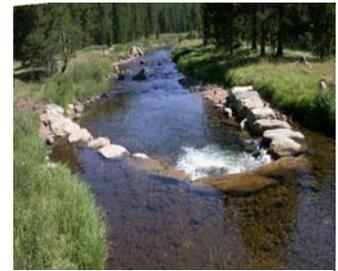
A “cross vane” structure is used to concentrate the flow of water down the middle instead of along the bank. This helps to alleviate bank erosion but also helps to create pool habitat for fish.
