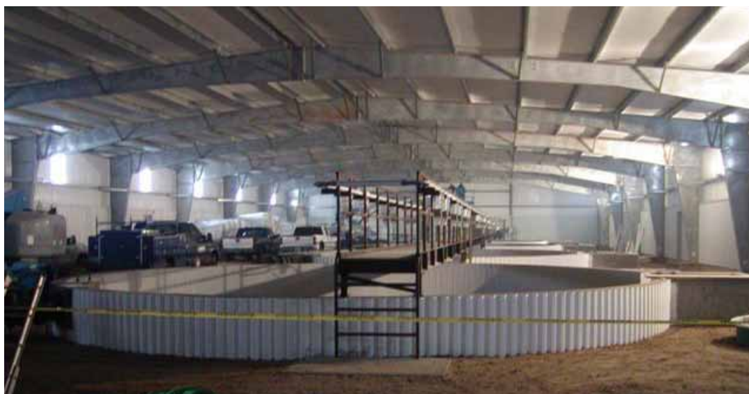
New 36 foot concrete circulars at Speas, there are now 8 total at Speas
