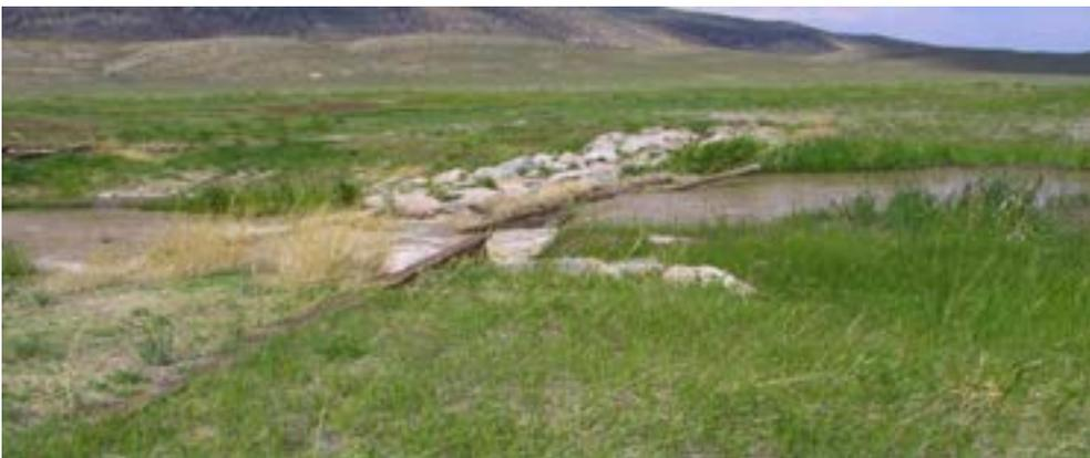
Drop structure on Diamond Creek. Note accumulated sediment in lower right portion of photo that has begun growing vegetation. Sediment is periodically removed to enhance the life of these types of wetlands.
