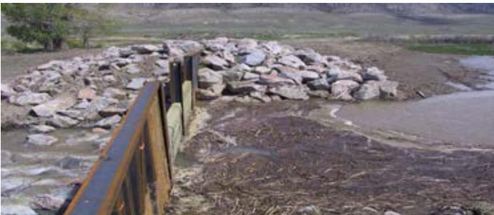
A new dike structure was completed in spring 2010 on Diamond Creek. It creates a five-acre wetland for sediment entrapment to prolong the life of Diamond Creek Dike Pond, a downstream Yellowstone Cutthroat trout fishery.
