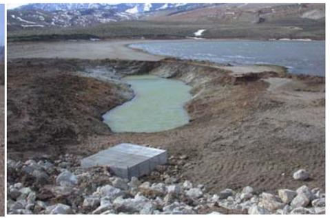
New outlet structure and removal of accumulated silt in Hogan Reservoir.
