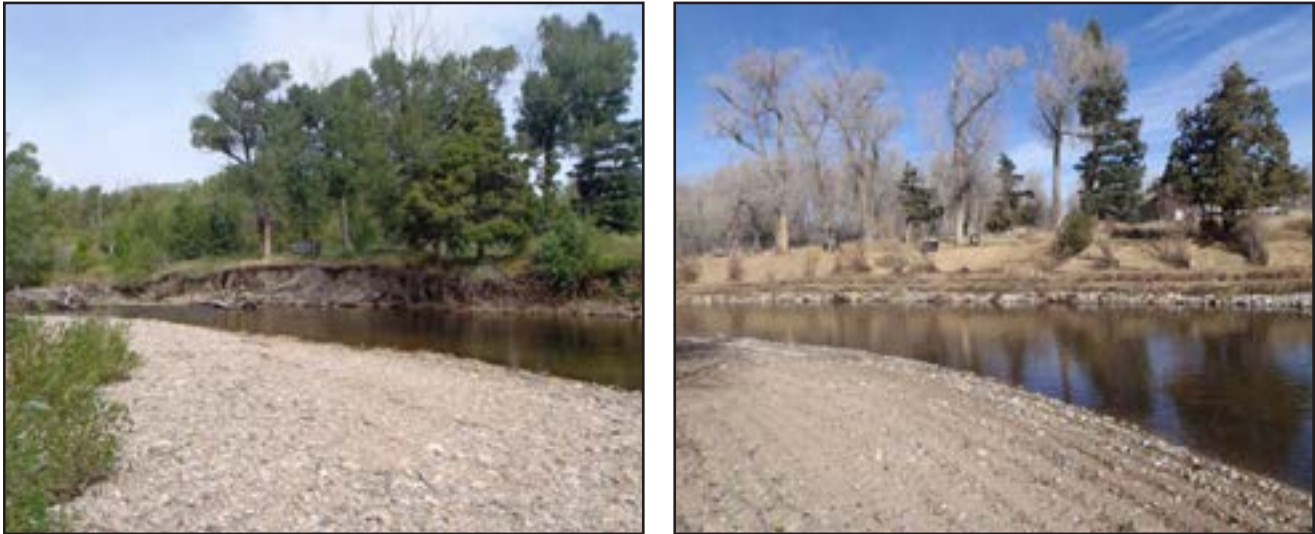
Figure 87. Encampment River - Richardson prior to bank stabilization (left) and following addition of toe wood, sod mats, willow clumps, and adjustments to bank angle (right).
