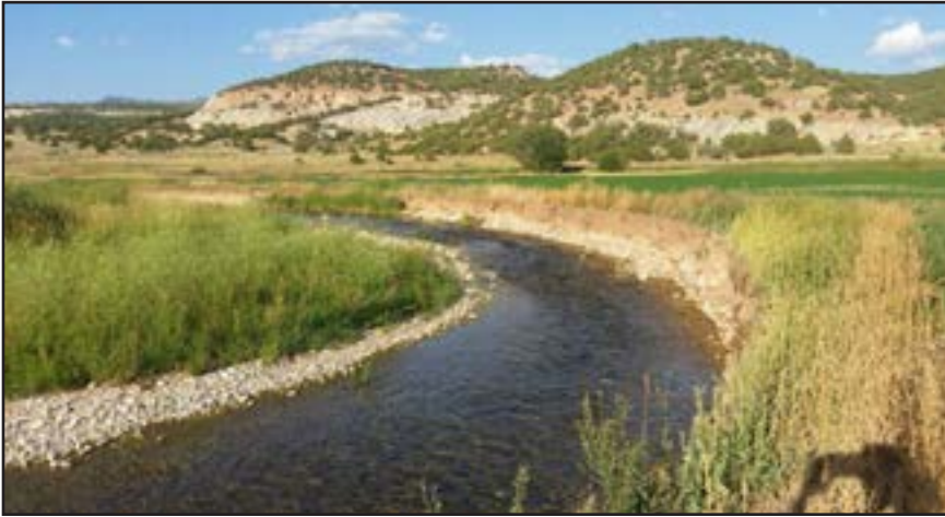
Figure 36. Lateral channel migration into a WGFD agricultural field and severe bank erosion. Stream bank is approximately 5-feet high.
