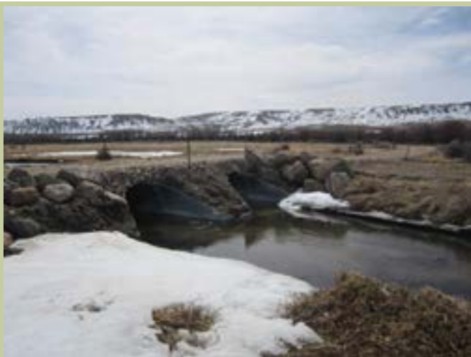
Figure 140. New culverts at Airport PAA.
