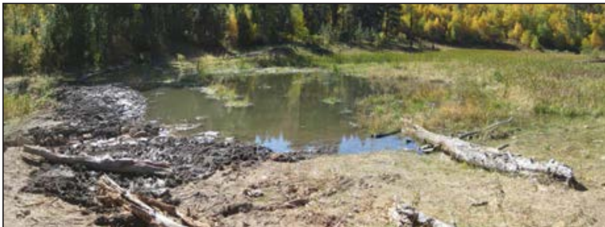
Figure 167. Grade control sill and floodplain bench to stop channel down-cutting and enhance a relic beaver dam wetland complex on Middle Redwater Creek.
