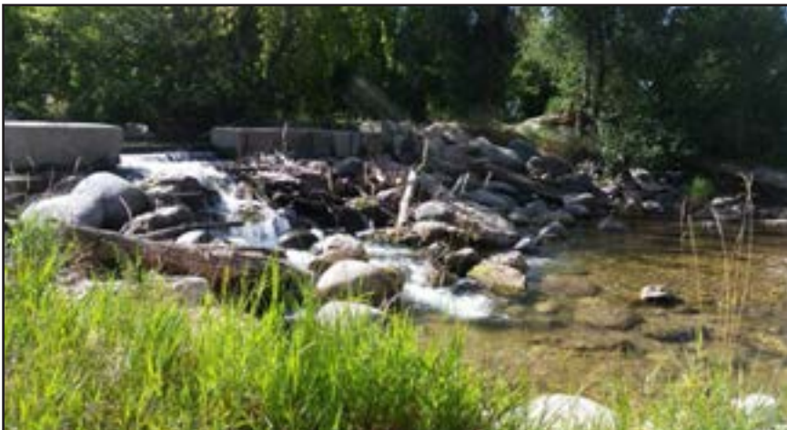
Figure 37. Downstream side of Anthony Diversion. The diversion dam is approximately six feet high and is a sediment and fish passage barrier.
