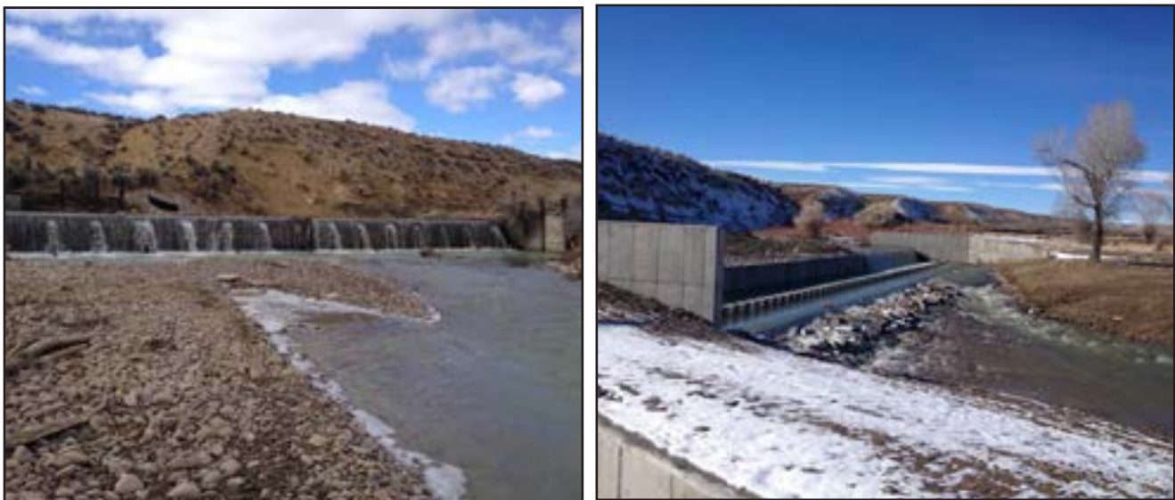
Figure 6. People’s Canal irrigation diversion pre (left) and post construction (right).
