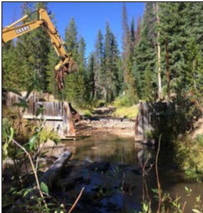
Figure 105. Removing hydrology weir from the East Fork Encampment River.
