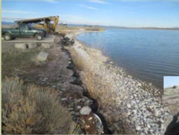
Figure 68. Geotextile fabric and rock (right) were added to the shoreline in the Long Point area within Ocean Lake WHMA (top)
