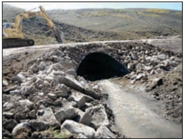
Figure 131. Bottomless arch-plate bridge structure installed over Coal Creek.
