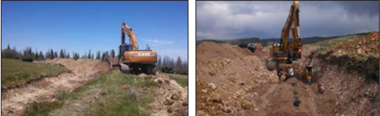
Figure 89. Heward Ditch pipe installation and screening.
