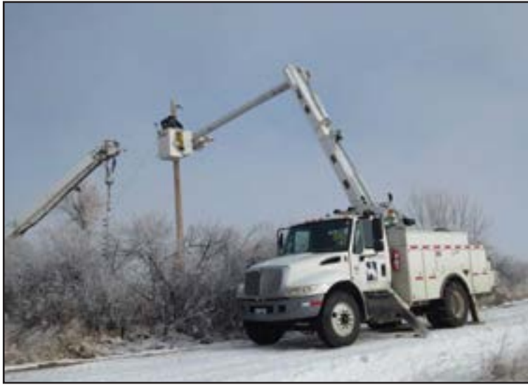
Figure 99. Table Mountain power line installation.
