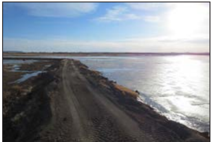
Figure 113. Table Mountain Dike Maintenance.
