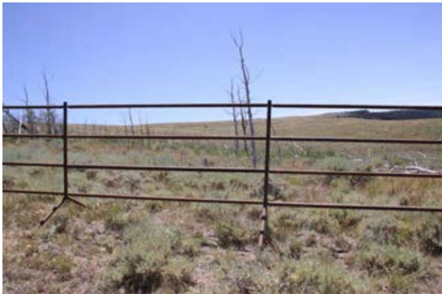
Figure 53. Modified Steel Jack Fence erected around an imperiled aspen stand.
