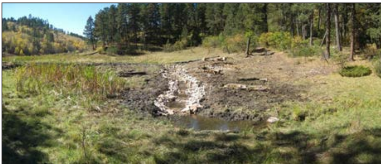
Figure 168. Step pool transition from a wetland complex to Middle Redwater Creek.
