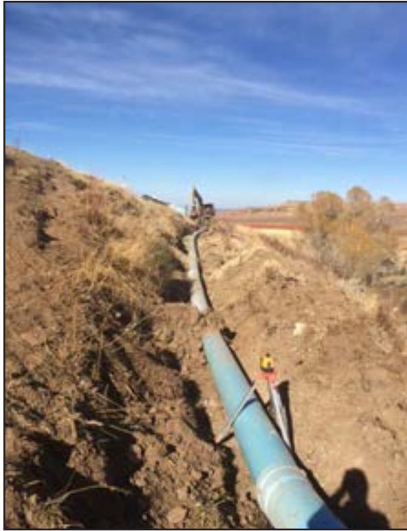
Figure 84. Installation of transport pipe.
