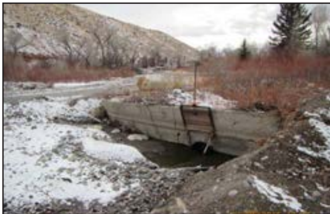
Figure 3. Condition of the old headgate that will be re-moved in fall 2016.
