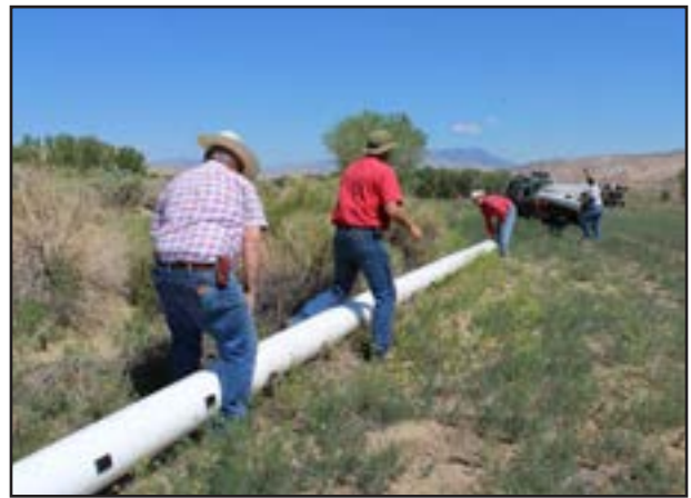
Figure 40. Gated pipe being placed on Yellowtail WHMA.
