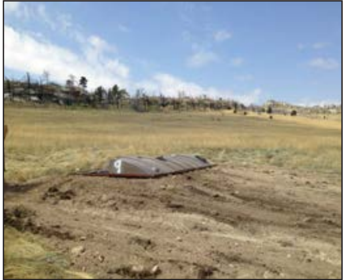
Figure 165. Installed 1,500 gallon BOSS watering tank.
