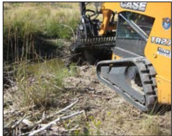
Figure 14. Skid steer used to place shredded tree material into Bolton Creek.
