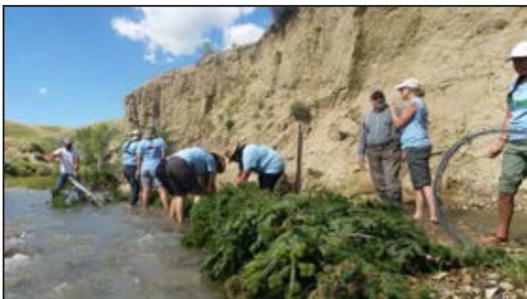
Figure 29. Volunteers installing tree revetments on Eaglenest Creek.
