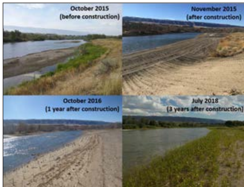
Figure 30. The Morad Park restoration site shows improvement in bank stability and riparian vegetation establishment. The bank was re-constructed to narrow the over-widened channel and to reduce the slope of the bank to reduce erosion potential. Willows and cottonwoods were planted to stabilize the new bank and were thriving by July 2018.
