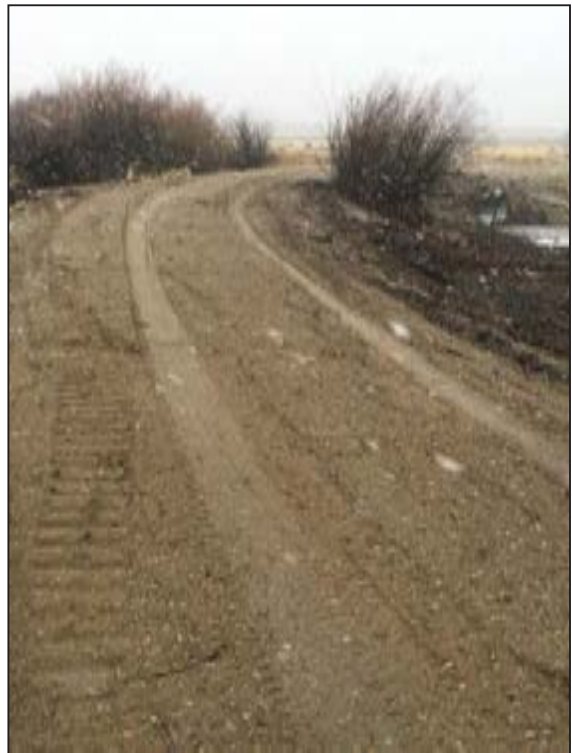
Figure 160. Access road repairs at New Fork River’s Airport PAA, Pinedale.
