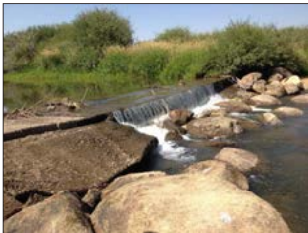
Figure 107. A diversion dam that is a barrier to most fish, but may be passable by trout.
