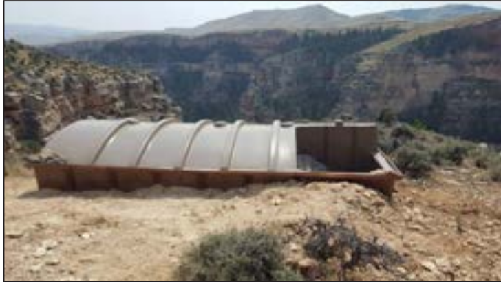
Figure 31. One of two guzzler tanks installed along the rim of Devil Canyon.
