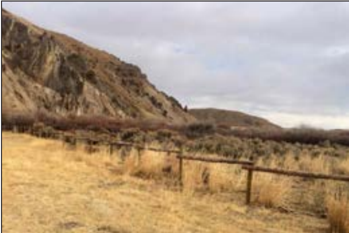
Figure 159. A fence that has been reconstructed to wildlife friendly specifications along LaBarge Creek. A pole top was included because this is in a riparian area and experiences significant use from moose.
