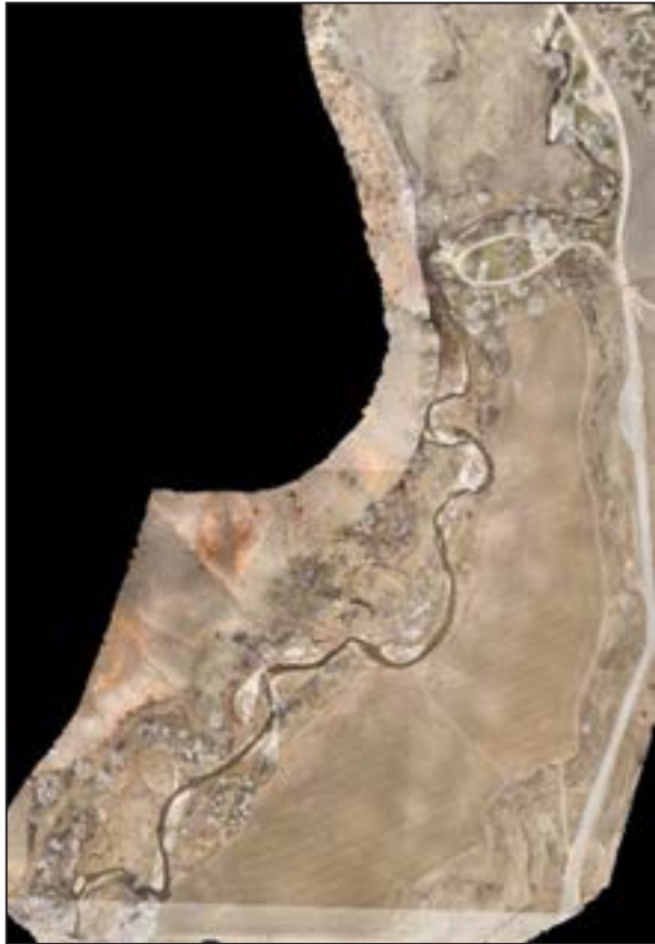
Figure 33. Aerial imagery of the pre-construction (October 2015) stream restoration area.
