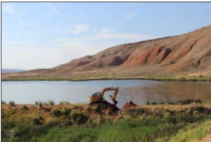
Figure 62. WGFD personnel breach Renner Reservoir dam.
