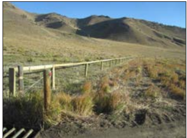
Figures 45-46. Newly constructed pole top boundary fence on the Sunlight WHMA.
