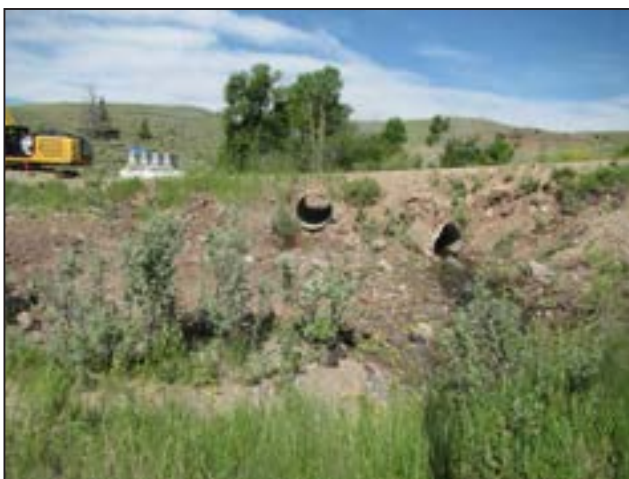
Figure 6. Crossing before construction.
