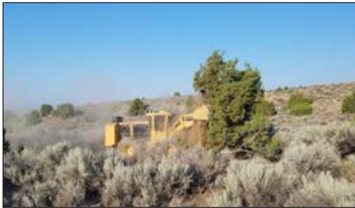
Figure 16. Juniper mulching with Tigercat equipment along Little Red Creek.
