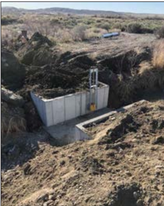
Figure 36. New concrete check and headgate.
