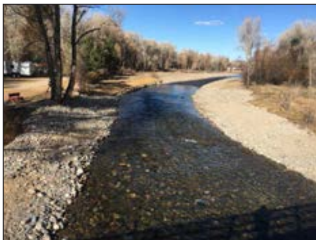
Figure 143. Looking downstream from Highway 230 bridge at the Encampment River after Riverside Phase 2 Restoration.
