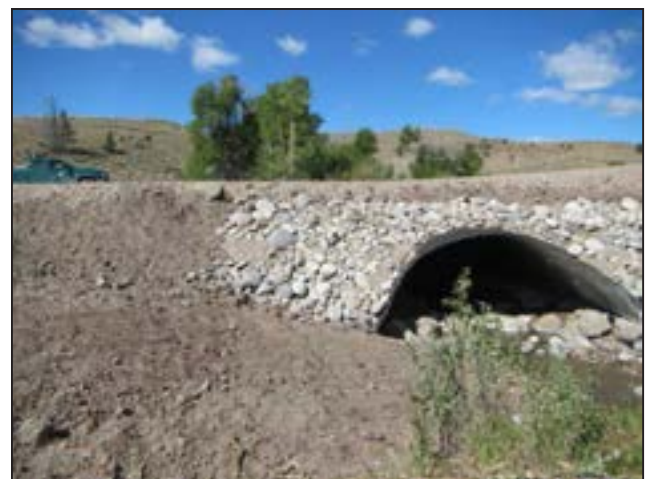
Figure 7. Crossing after construction.
