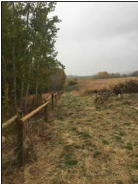
Figure 97. Coco Belle new wildlife friendly pole top fence.
