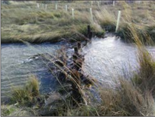
Figure 60. A BDA two years after installation on Eaglenest Creek. The green tubes are browse protection for shrub plantings.
