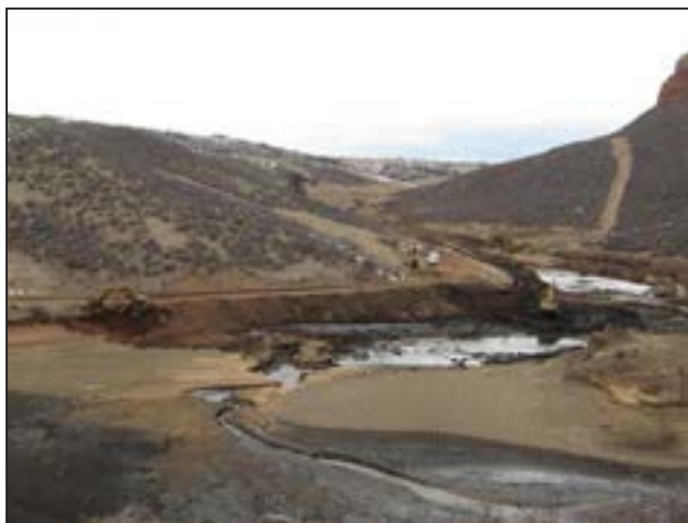
Figure 158. Lower North Crow Reservoir sediment removal.
