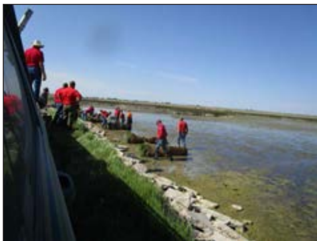
Figure 153. Vegetation mats being unrolled prior to staking at Table Mountain WHMA.
