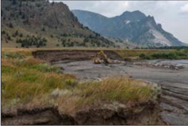
Figure 47. Sunlight Creek eroding bank prior to construction.
