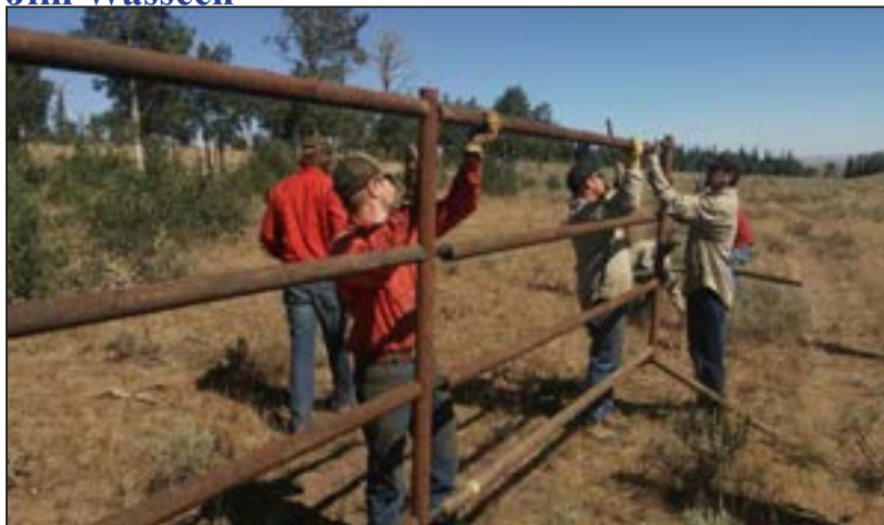
Figure 85. Partners erect phase III steel jack fencing on Little Mountain to protect aspen regeneration from overbrowsing.
