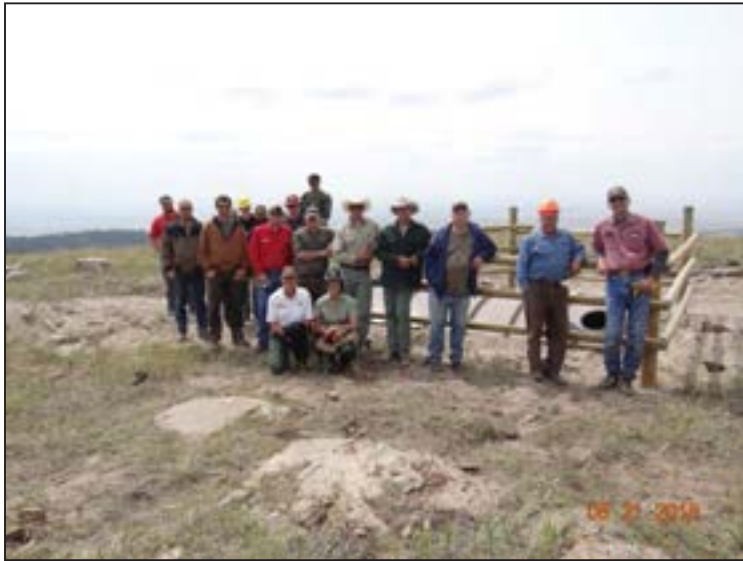
Figure 24. Elk Mountain guzzler installation crew.
