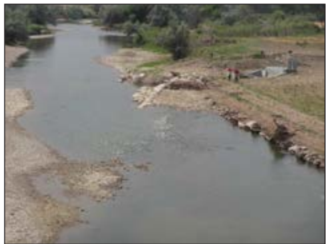
Figure 3. Overview of Harmony Diversion at its new location.
