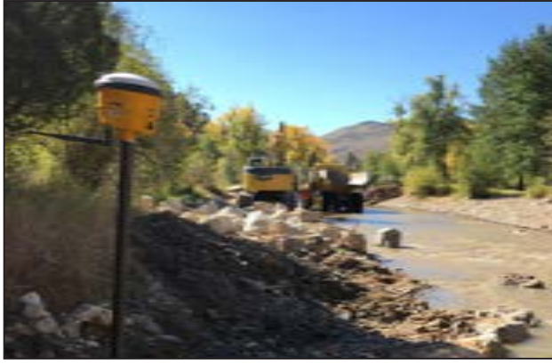
Figure 144. Constructed riffle on Encampment River-Pickett Restoration.
