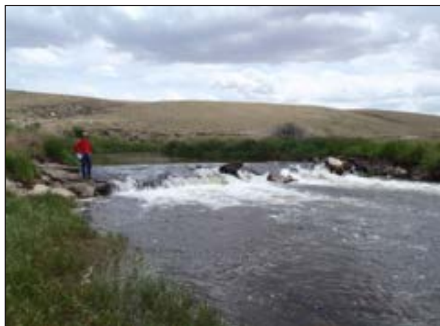
Figure 106. A diversion dam that is a barrier to fish passage.
