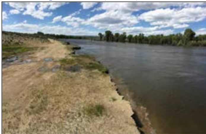
Figure 187. The “Gas Wells” site on the New Fork River historically supported a boat ramp, but has been lost in recent years due to lateral migration of the river channel.
