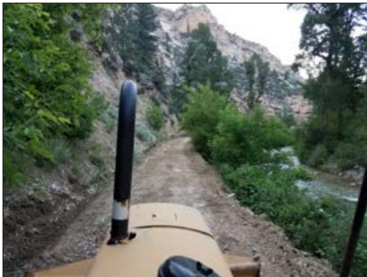
Figure 203. A bulldozer was required to re-shape and grade Kerns WHMA access road to reduce erosion and improve public access.
