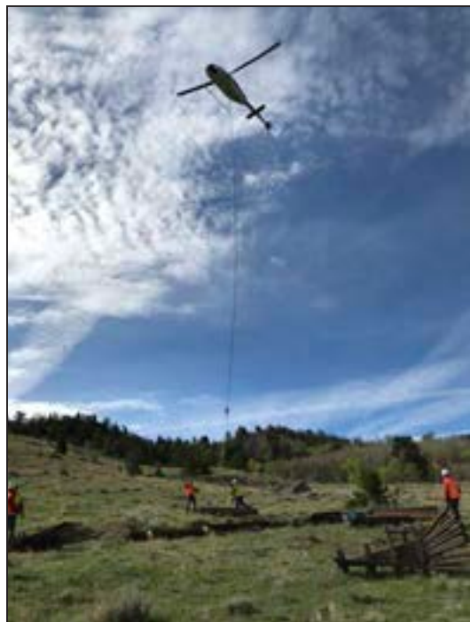
Figure 123. Drill stem pipe fencing materials being aerially delivered to a spring location on Green Mountain. The fence will protect a spring from overuse by livestock, feral horses and wildlife.
