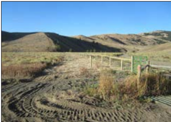
Figures 45-46. Newly constructed pole top boundary fence on the Sunlight WHMA.
