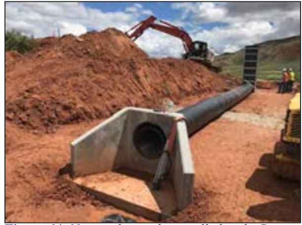
Figure 64. New outlet works installed in the Renner Reservoir dike.
