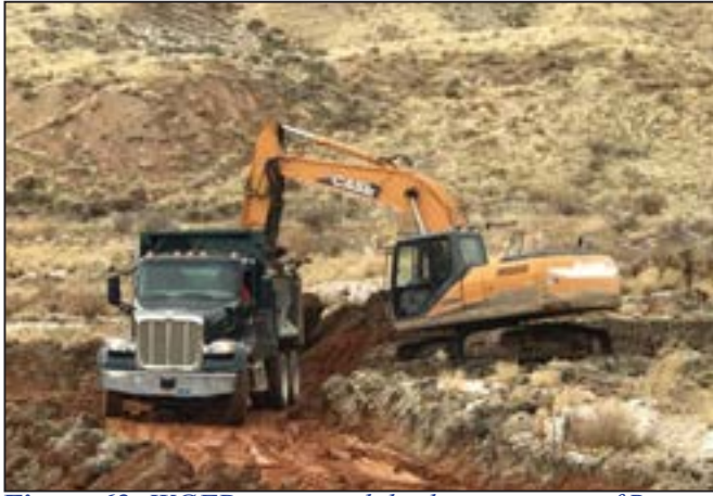
Figure 63. WGFD personnel dredge a portion of Renner Reservoir.
