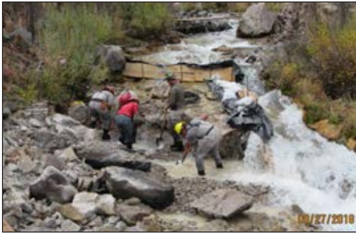
Figure 5. Debris being cleared on Sheridan Creek post-blasting to create a fish barrier.
