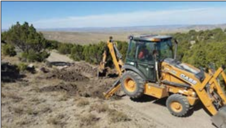
Figure 73. Access road repairs on Hank's Hill at Bear River PAA.
