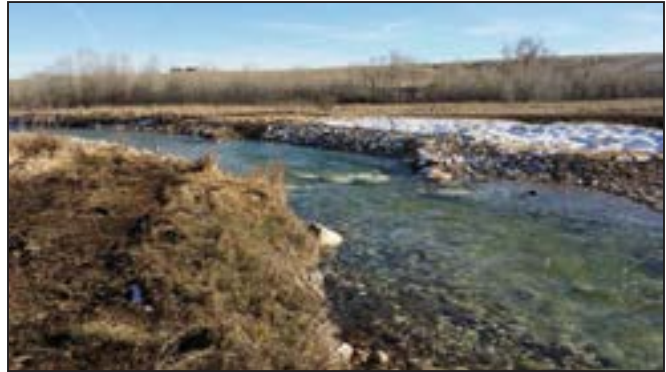
Figure 208. Vane and bankfull bench treatments on the Tongue River above Dayton, WY.
