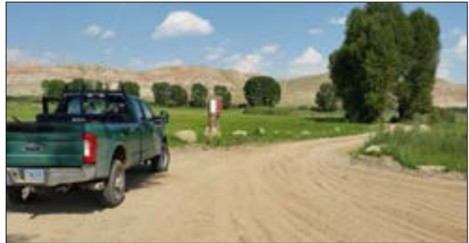
Figure 158. Parking area and access road repairs at Green River Fear access.
