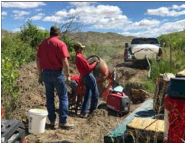
Figure 23. Personnel mixing concrete for the diversion box.
