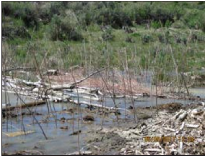
Figure 14. Willow stakes placed in sediment.
