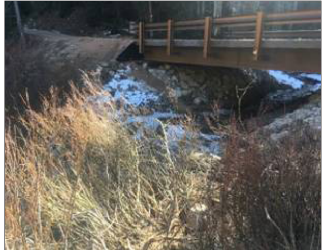
Figure 2. Crystal Creek after bridge installation.
