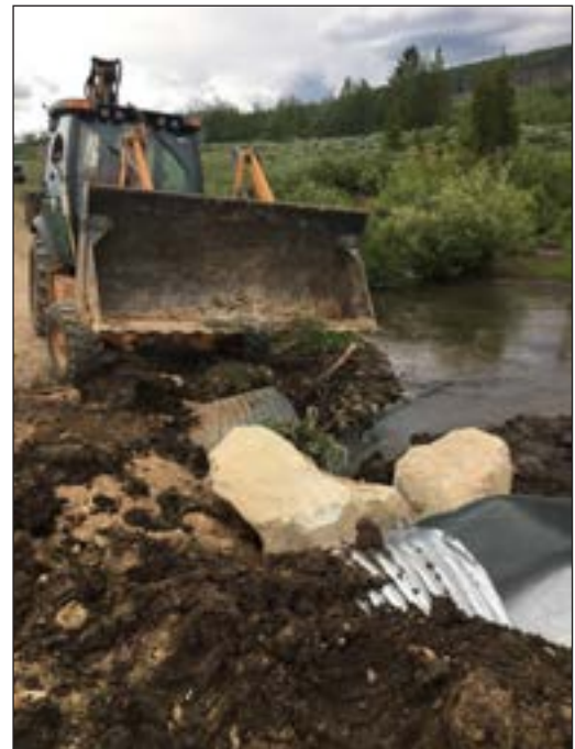
Figure 62. Road maintenance on Minnie Holden Creek to access V-Cross PAA.
