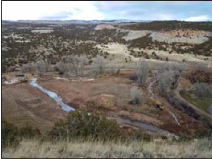
Figure 32. Overview of the new Medicine Lodge Creek channel. The State Park Bridge is visible in the upper left and rock drop structures that replaced the Anthony Diversion are on the right.
