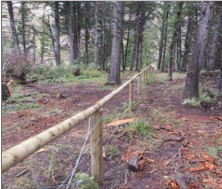
Figure 27. Newly constructed wildlife friendly pole-top fence on Medicine Lodge WHMA.
