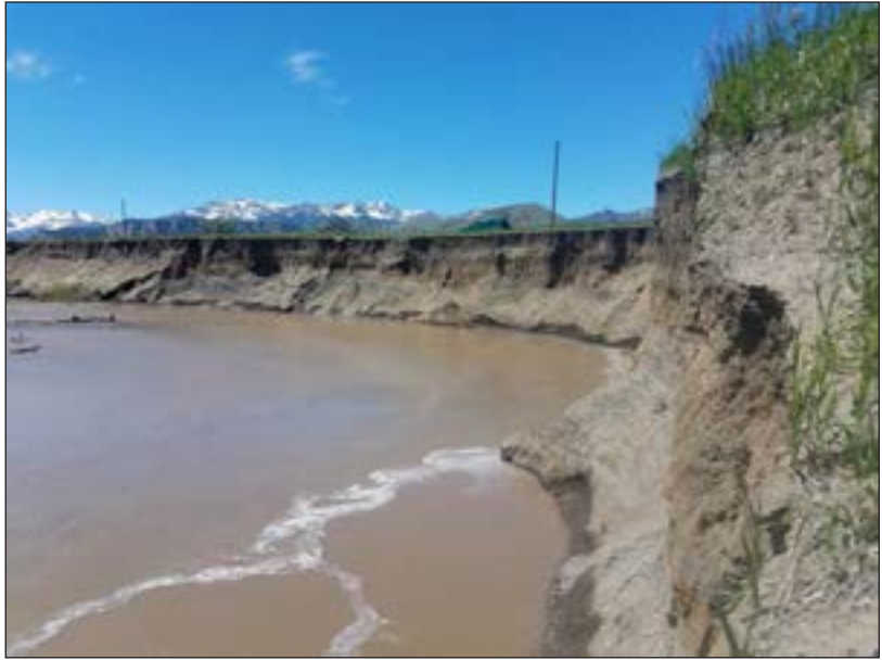
Figure 42. Sunlight Creek after 100-feet of lateral erosion during 2017 spring runoff.
