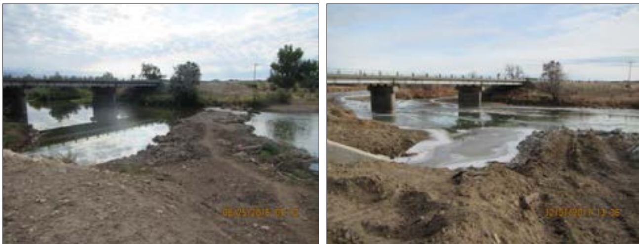
Figure 11. Before (left) and after (right) removal of the old diversion dam downstream of the Highway 31 bridge.
