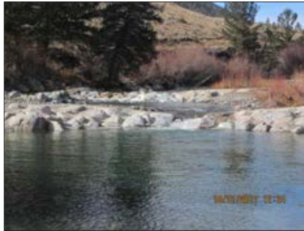
Figure 6. Lower rock ramp after construction.
