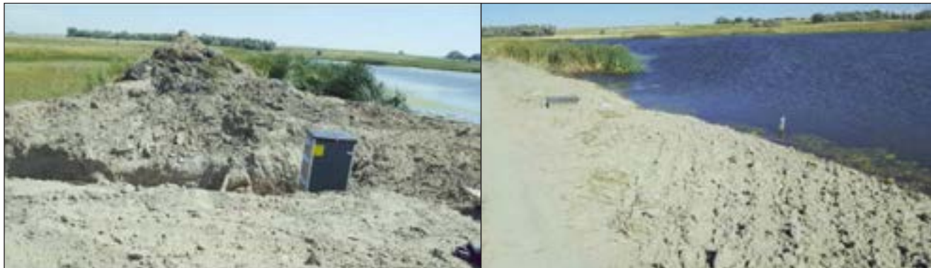
Figure 122. Agri-Drain being installed (left) and after installation (right). Photo courtesy DU.
