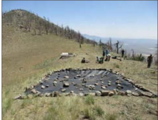
Figure 98. Catchment apron and guzzler installed on Garden Creek.
