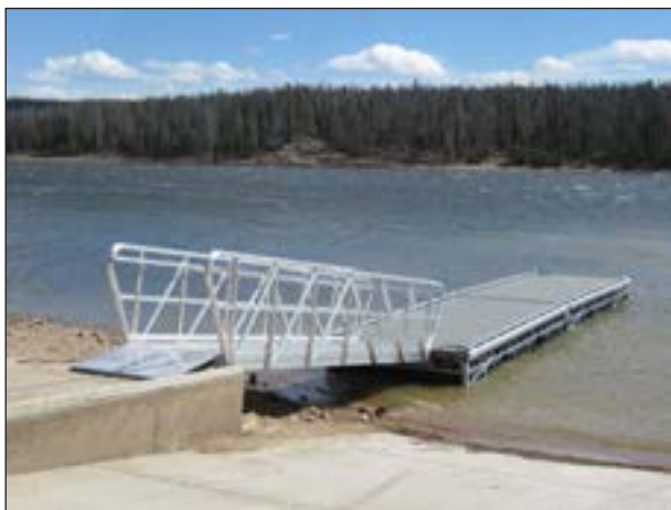
Figure 118. Boat dock replacement.
