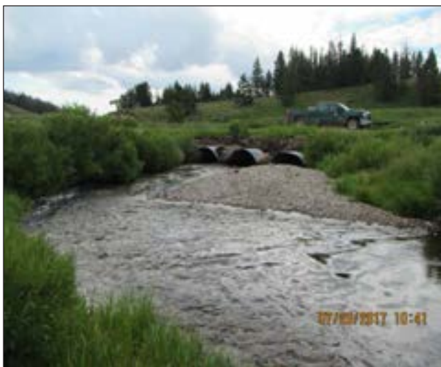
Figure 3. Big Warm Springs Creek Crossing before construction.
