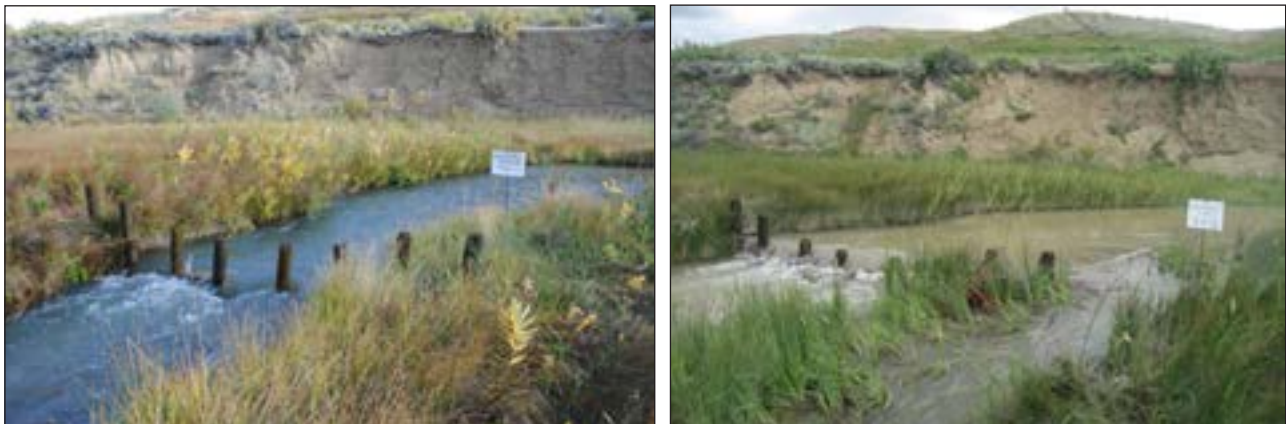
Figure 38. 2016 during construction of a BDA (left) and 2017 during high flow (right).
