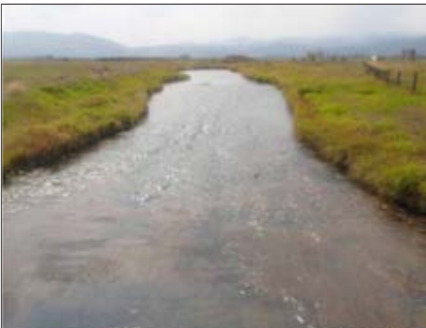
Figure 73. Channelization and willow removal yielded an overly-wide and shallow Flat Creek channel.
