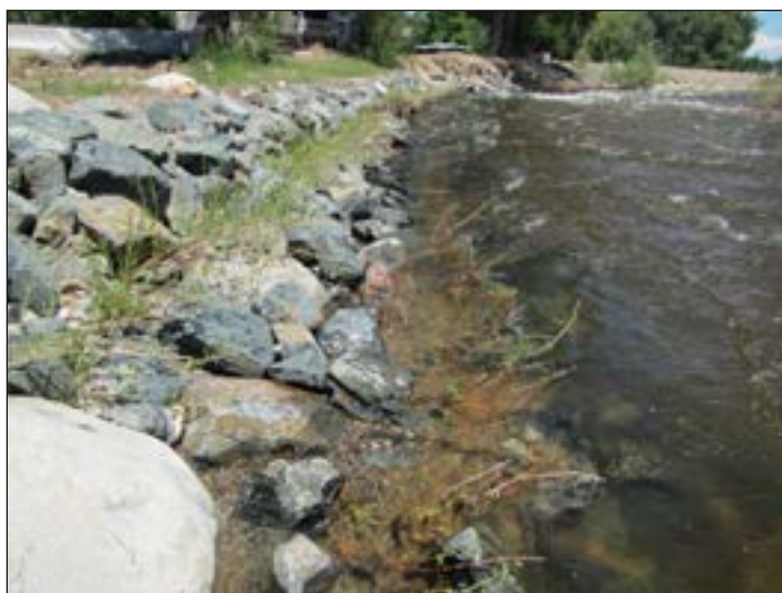
Figure 80. Rock and willow bank stabilization during 2017 runoff.
