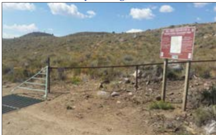
Figure 161. Wildlife friendly pipe fence on Fall Creek WHMA.
