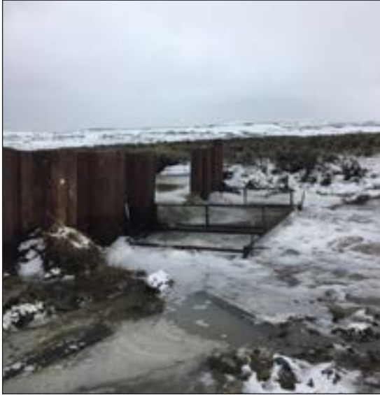
Figure 53. Fish screen installation on Sculpin Creek.
