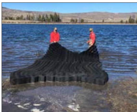
Figure 127. Geoweb ramp installation at Dollar Lake.
