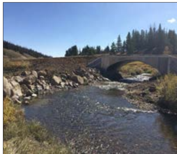
Figure 4. Big Warm Springs Creek crossing after construction.
