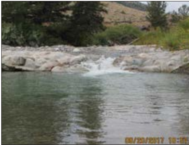
Figure 5. Lower rock ramp since 2014 and prior to construction.
