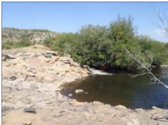
Figure 116. Big Creek Diversion before fish passage construction.
