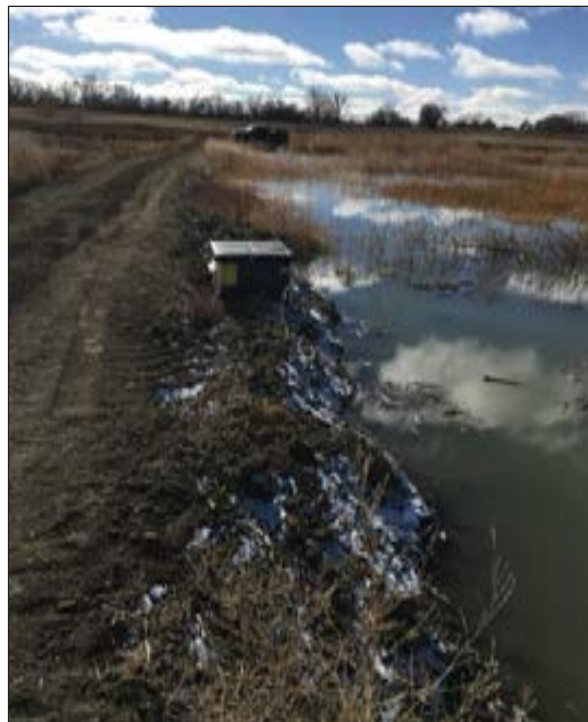
Figure 96. Flooding of new wetland.
