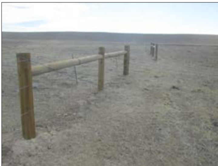
Figure 107. Completed section of wildlife friendly fence. Photo credit Medicine Bow Conservation District.
