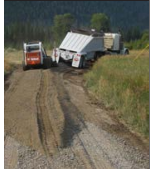
Figure 25. Roadbase being spread and bladed on Sunlight WHMA.
