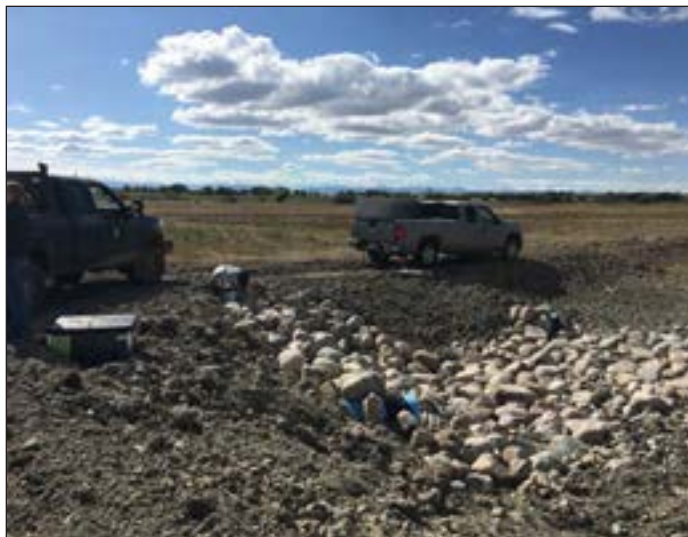
Figure 95. Newly constructed water control structure.
