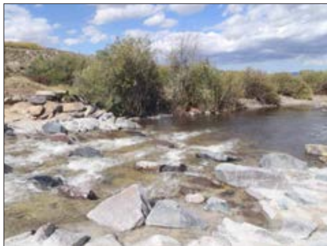
Figure 117. Big Creek Fish Passage rock ramp fishway after construction.
