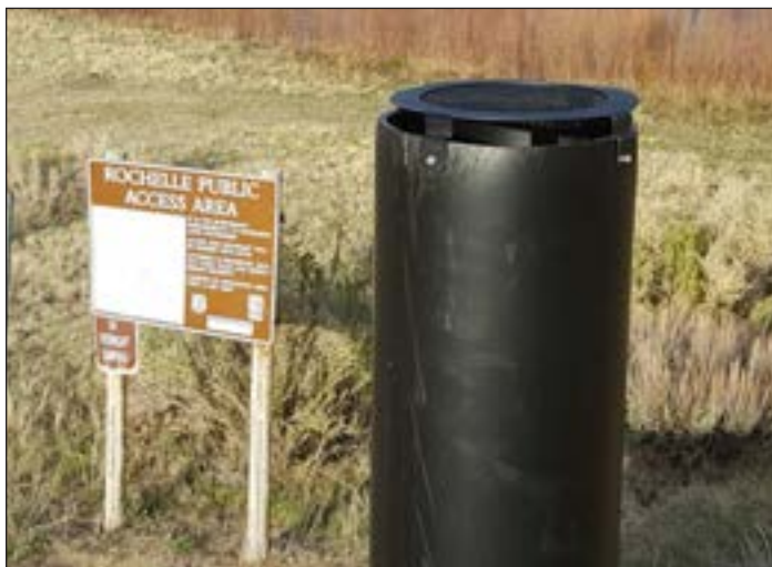
Figure 111. Comfort station vent covers.
